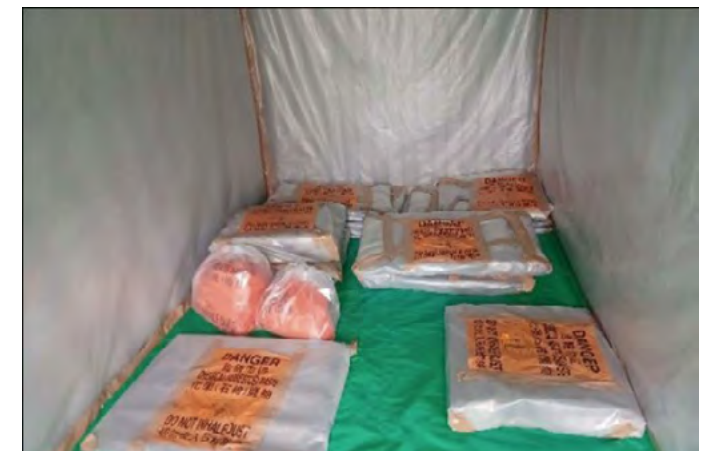
石棉廢物袋（核准尺寸為1米×0.7米、承載能力為兩公斤） Waste bags with approved size of 1m x 0.7m and loading capacity of 2kg
