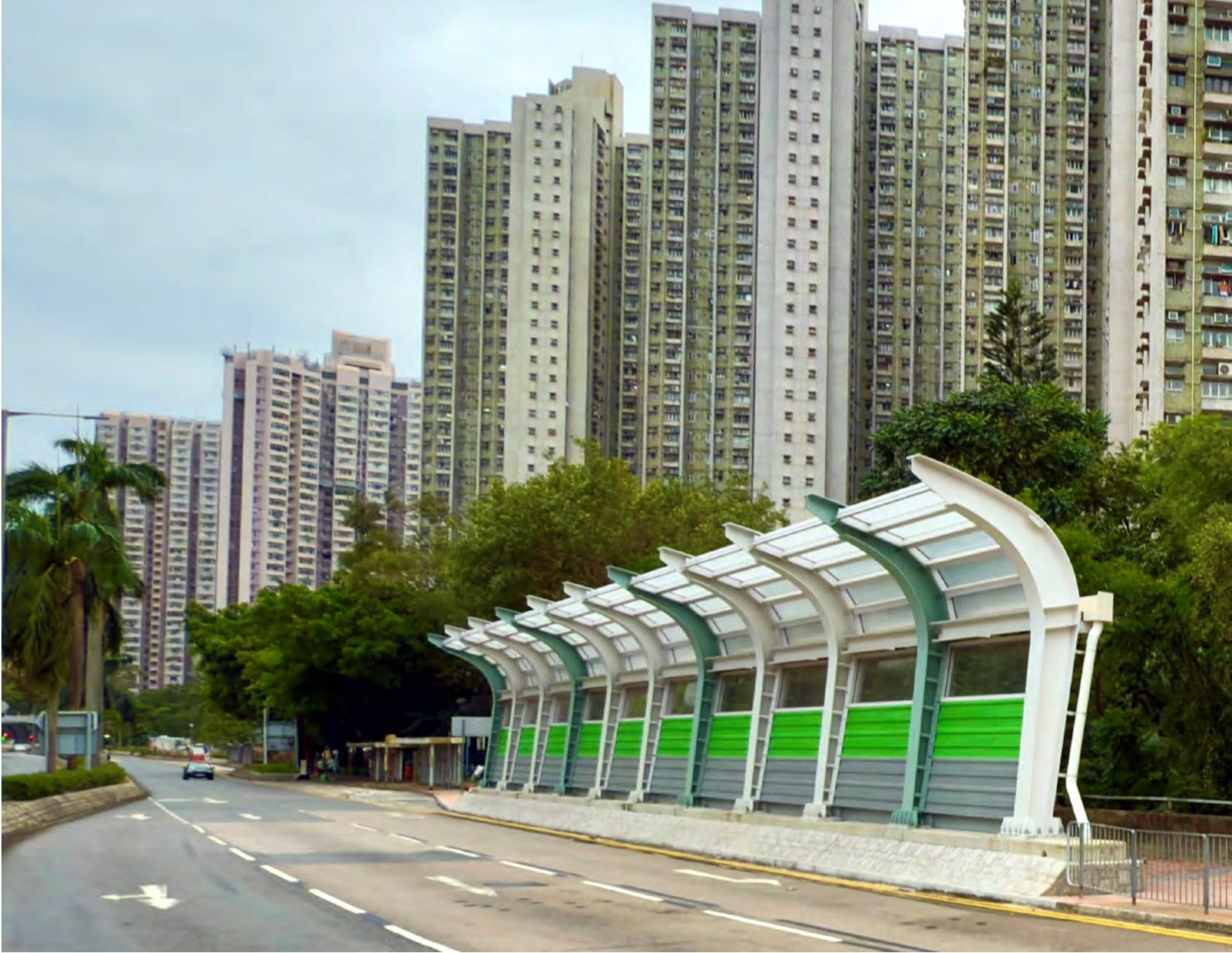
在懸臂式隔音屏障應用 S690 高強度鋼材 Application of S690 high-strength steel on cantilevered noise barrier
