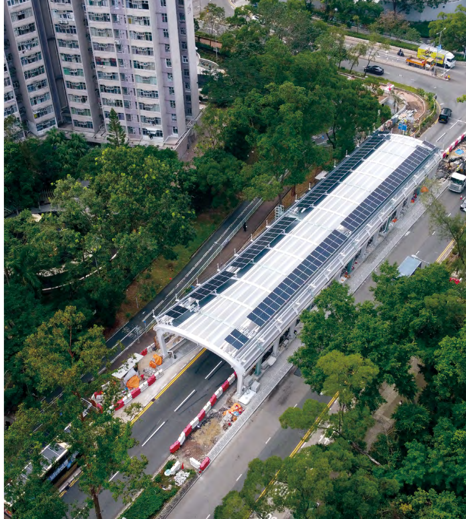
在隔音罩安裝光伏系統 Installation of PV systems on noise enclosure
