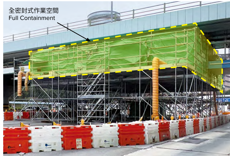
為移除含石棉物料簷篷而設立的全密封式作業空間 Full containment for ACMs contained canopy removal
