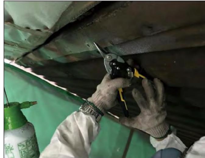
以手工工具配合噴霧移除金屬殼 Trimming of metal cladding by hand tools with water spray
