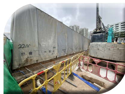
豎設隔音屏障
