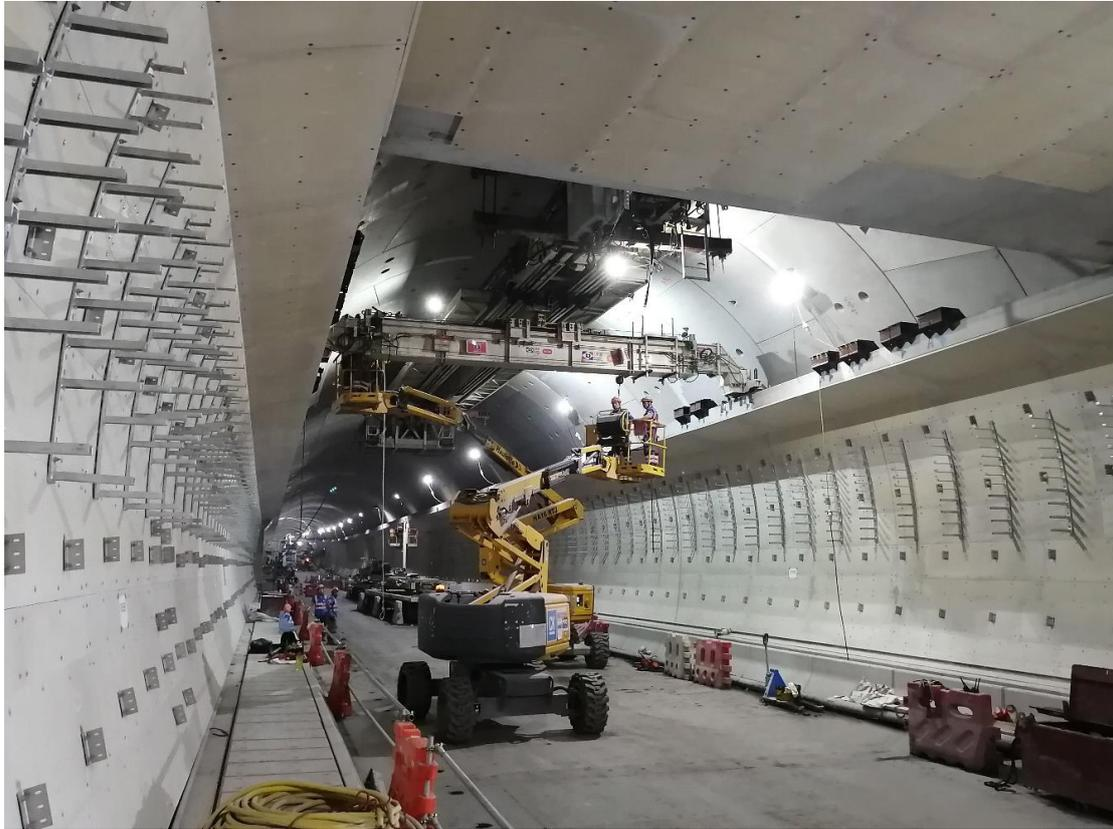
*在隧道內組裝架空通風管預製面板*
