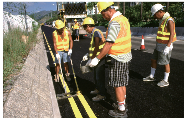
重髹道路标记 Road marking repaint
