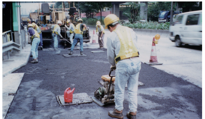
在快速道路上铺设承重层 Laying of base course on in High Speed Road
