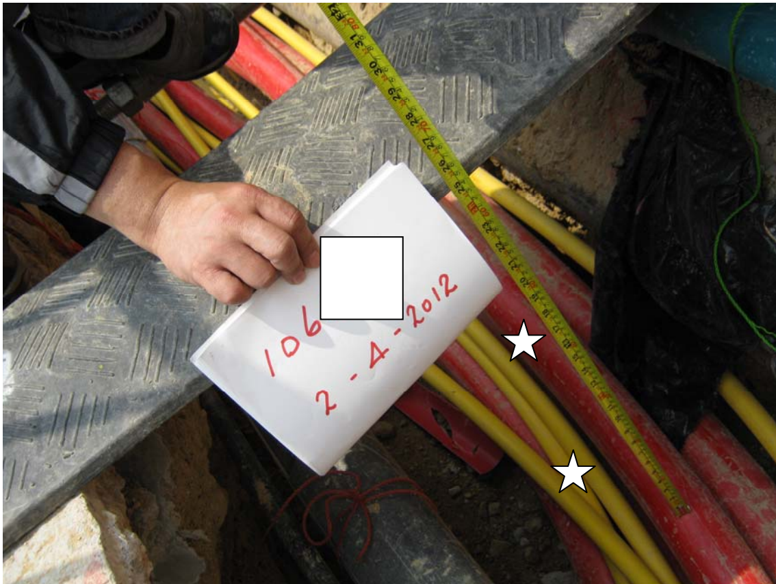
Photo 3B (Depth of Services/Installation = 640mm)
