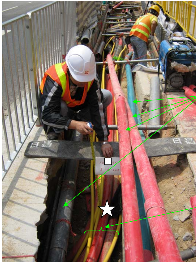
Photo 3A (Depth of Services/Installation = 640mm)
