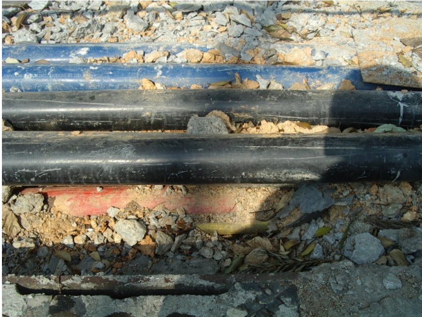
Photo 1 – PVC Duct (NWT)
