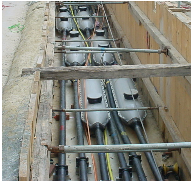
132kV Cable & Joint
