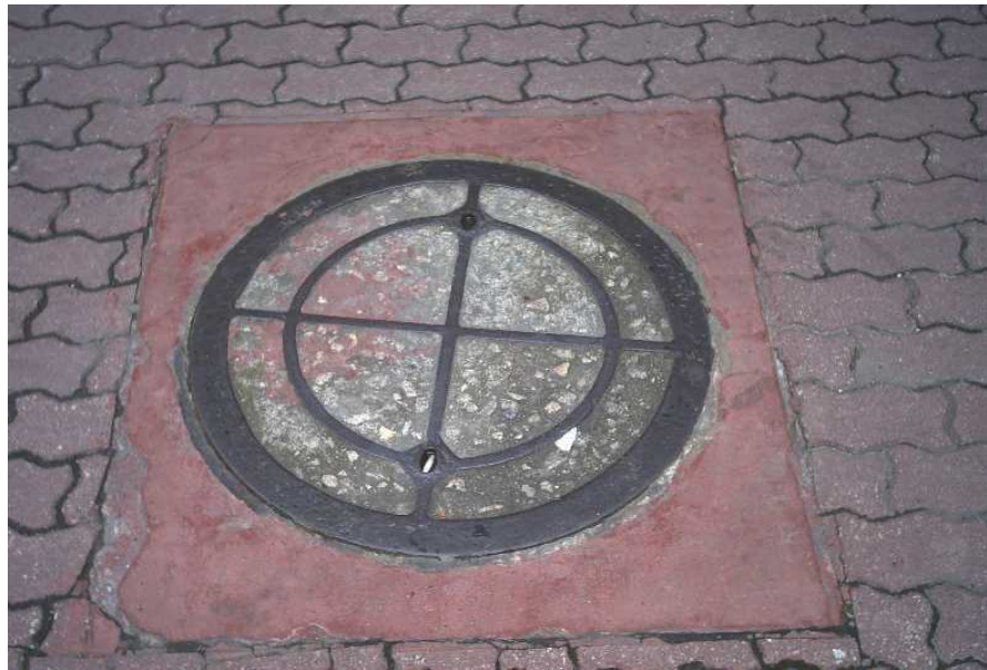
Photo No. 11 (Manhole – Carriageway Type) Circular Cover
