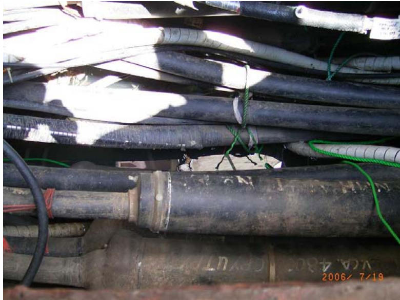
Photo No. 5 (Cables)
