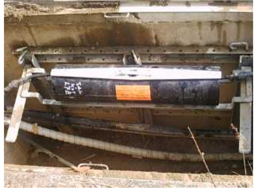
Photo No. 6 (Cable Joint)
