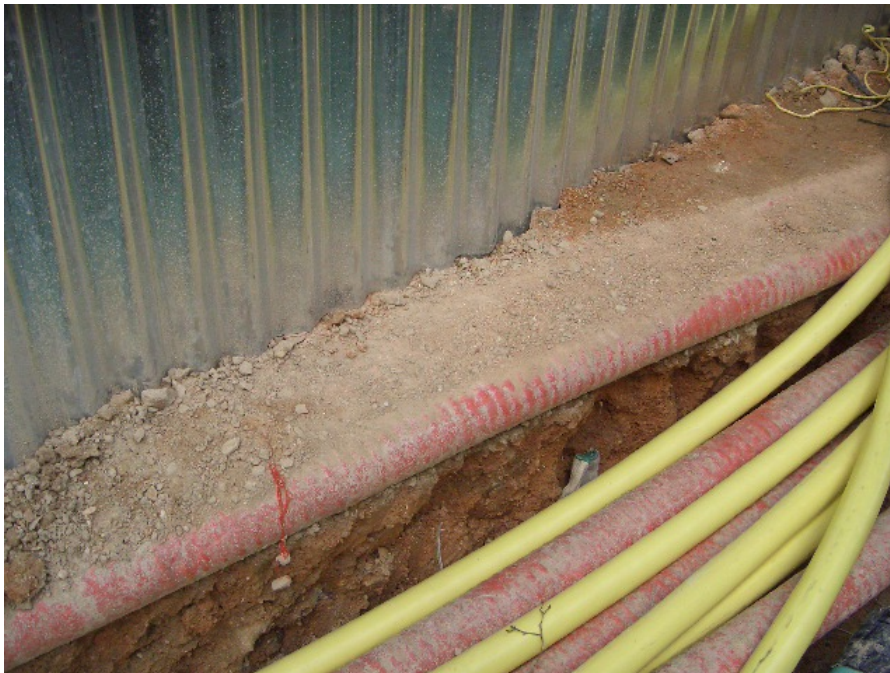
Photo 2 - 11kV Cables
