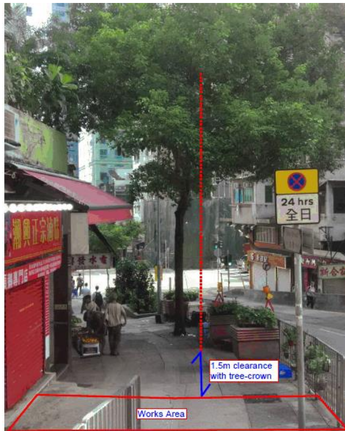
Photo 1: Vertical clearance between tree-crown and works area
