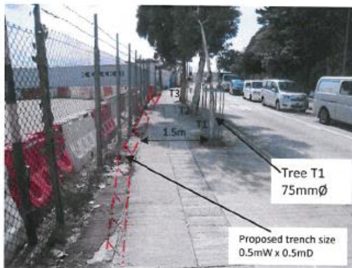
Photo 1: Horizontal clearance between trees and works area (with trees' diameter at breast height)
