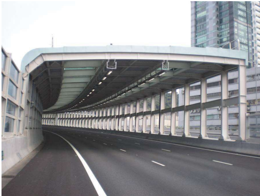
Figure F8 – Noise semi-enclosure at Lai Chi Kok viaduct (Route 8) (Vertical part: Transparent panels; Roof: absorptive panels and transparent panels)
