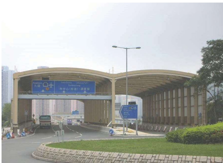
Figure F10 – Noise enclosure designed to enclose a sign gantry
