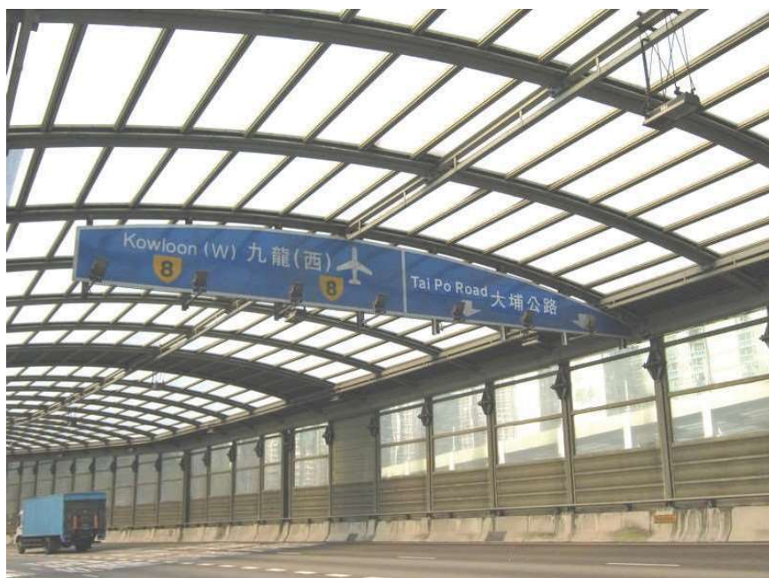
Figure F12 – Directional signs designed to suit the profile of the noise enclosure roof
