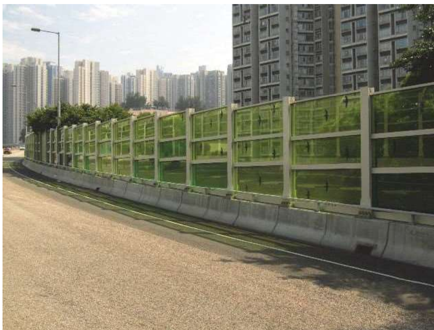
Figure F5 – Vertical noise barrier at Kwun Tong Bypass (Transparent panels)
