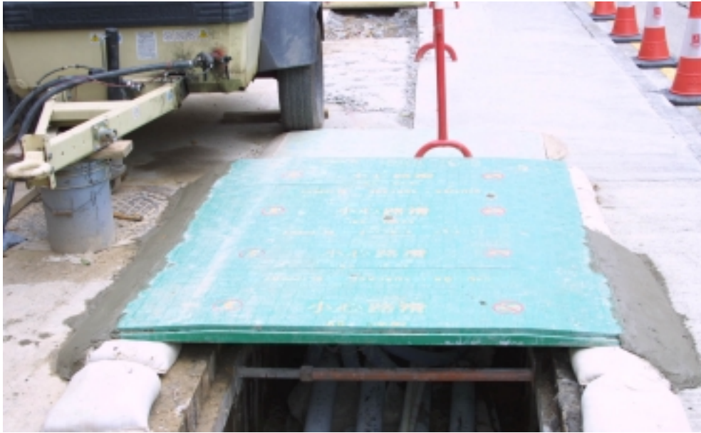
Plate B3 – Sandbag upstand with fibre-glass cover to prevent surface runoff and infiltration of rainwater
