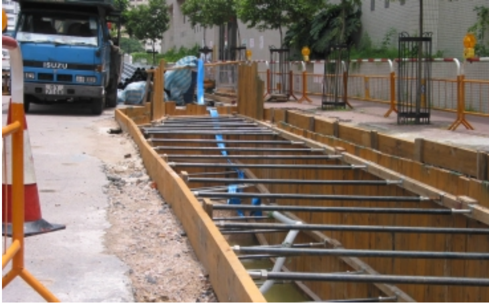
Plate A3 – Timber support for deeper excavation
