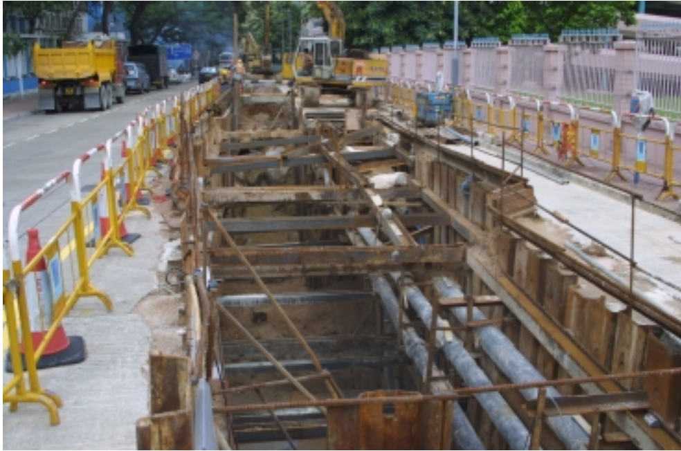
Plate A5 – Steel sheet pile support
