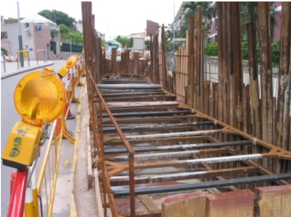
Plate A4 – Steel sheet pile support
