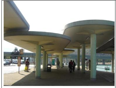
Bus shelter with reinforced concrete cover:
