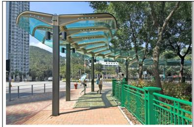
Walkway cover with transparent panels spanning over full walkway width and high headroom:
