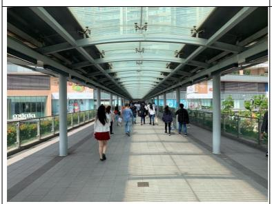
Footbridge with hybrid cover (about one-third of width with transparent panels and two-third of width with opaque panels):
