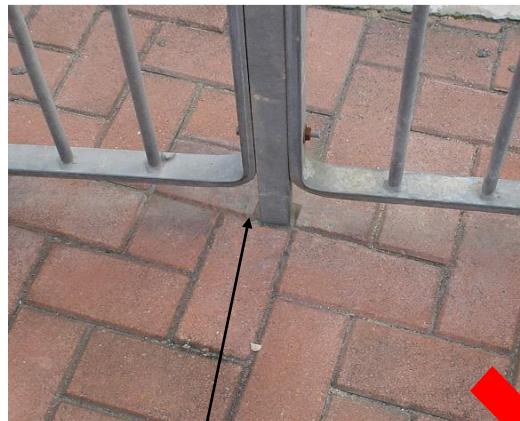
Footing should be recessed and cut blocks to fit
