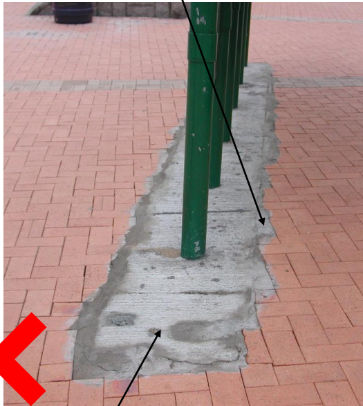
Existing exposed footing
