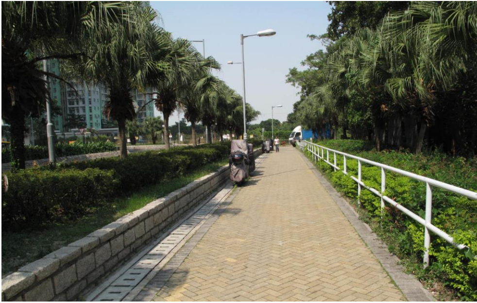
Plate 4.2 – Using smaller paving units on narrow footway
