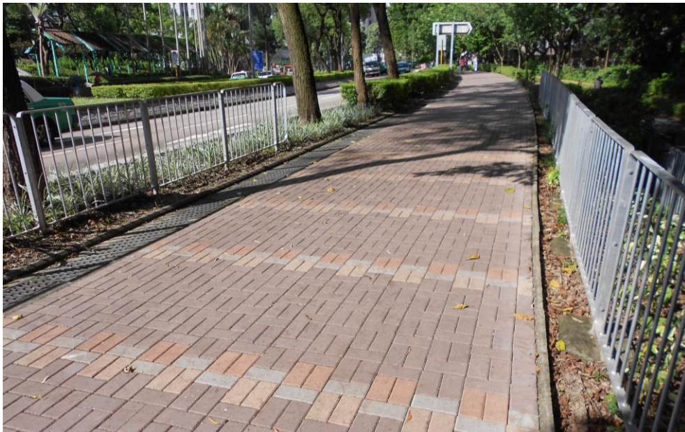
Plate 4.11 – Using a simple texture and uniform laying patterns along a localized strip of pavement
