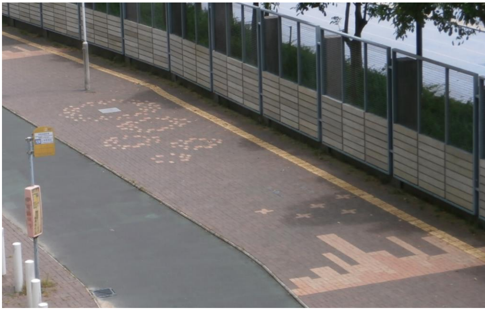
Plate 4.8 – Using an elaborate laying pattern design
