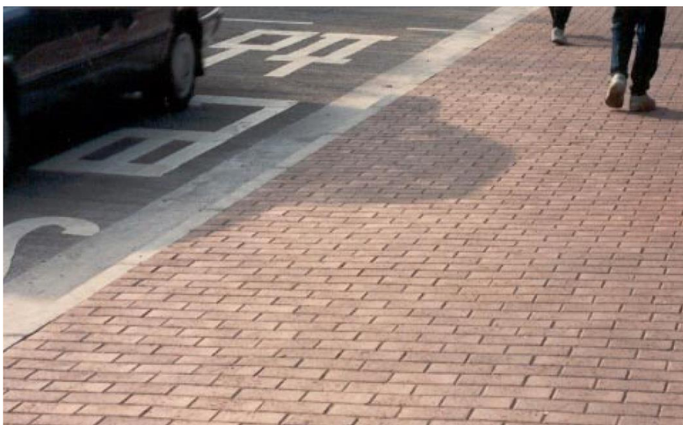
Plate 4.5 – Using rectilinear laying pattern to align with straight kerbside
