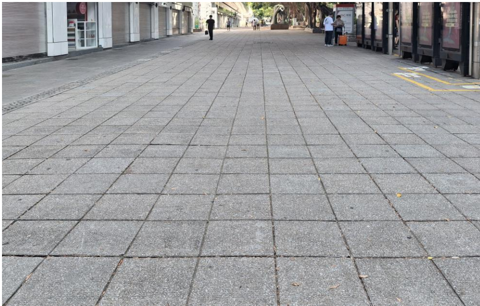
Plate 4.3 – Using larger paving units on wide footway
