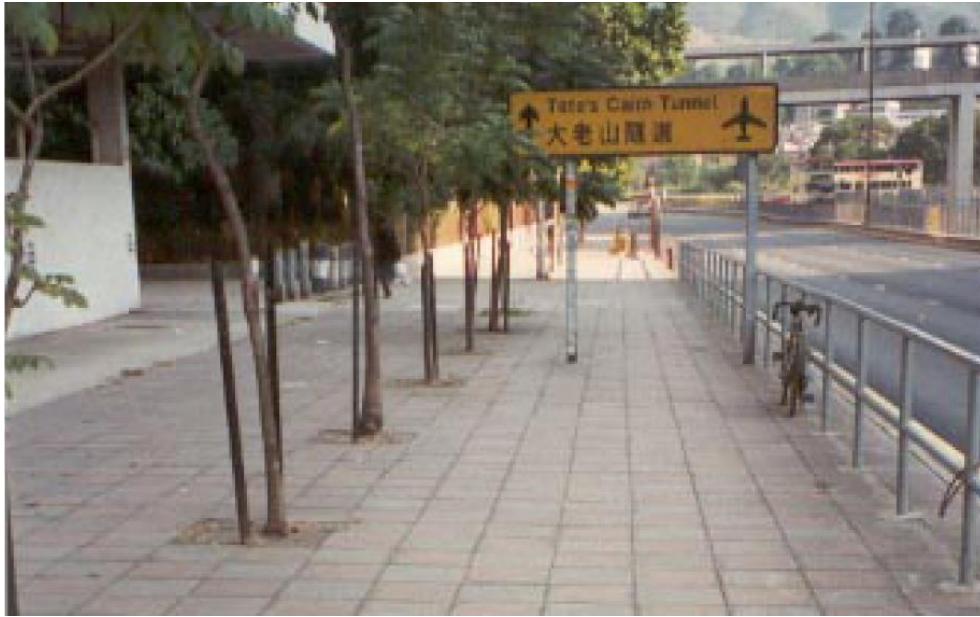
Plate 4.3 – Using larger-sized paving units on wide footway
