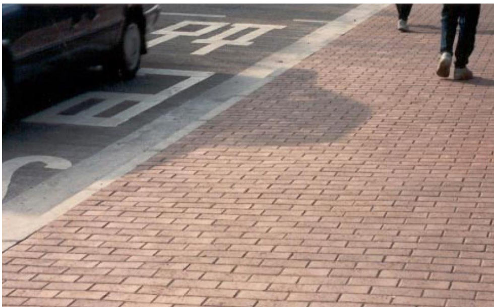
Plate 4.4 – Using rectilinear laying pattern to align with straight kerbside
