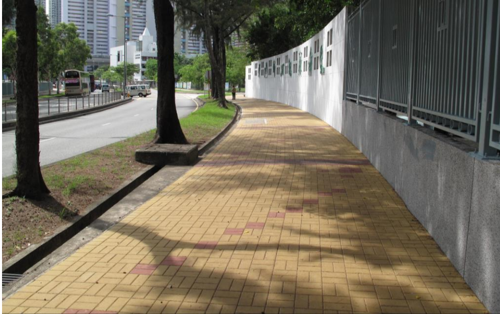
Plate 4.5 – Using transverse paving bands as transitional zones for aligning the direction of a laying pattern with the curvature of a footway to provide visual continuity
