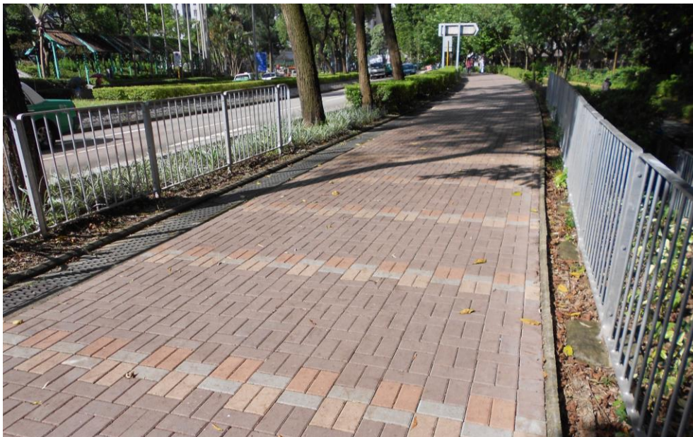
Plate 4.10 – Using a simple texture and uniform laying patterns along a localized strip of pavement
