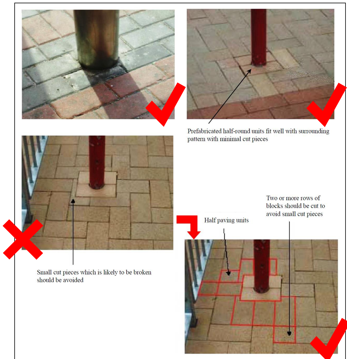
Figure 6.11 – Treatment to paving units around posts and columns
