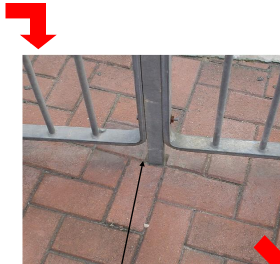
Footing should be recessed and cut blocks to fit
