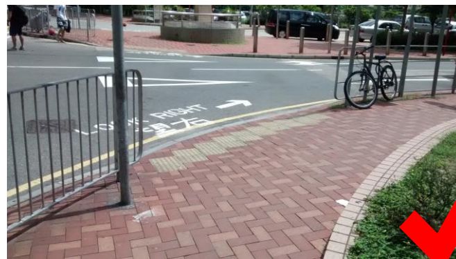
Good visual contrast between pavers and tactile warning strip
