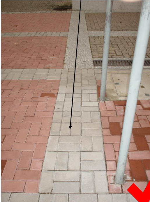
Use of banding at logical cut-off / change of materials
