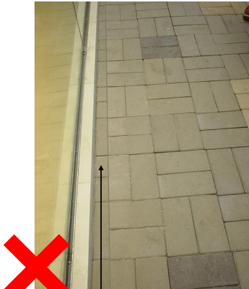
Poor practice for cut less than 1/3 of a block size
