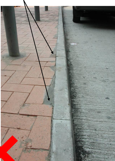
Unsightly concrete infill
