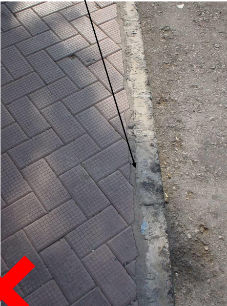
Untidy concrete infill due to irregular edge line of cut blocks
