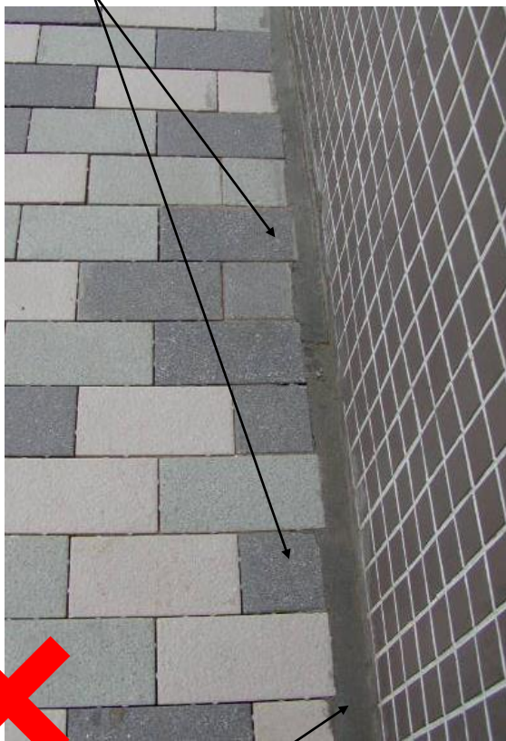
A wide gap with uneven concrete infill
