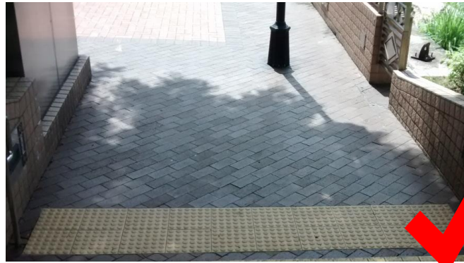
Good visual contrast between dark color pavers and yellow tactile warning strip
