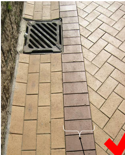
A dark brown band delineates ditch of stretcher bond on the left and footway of herringbone bond laying pattern on the right
