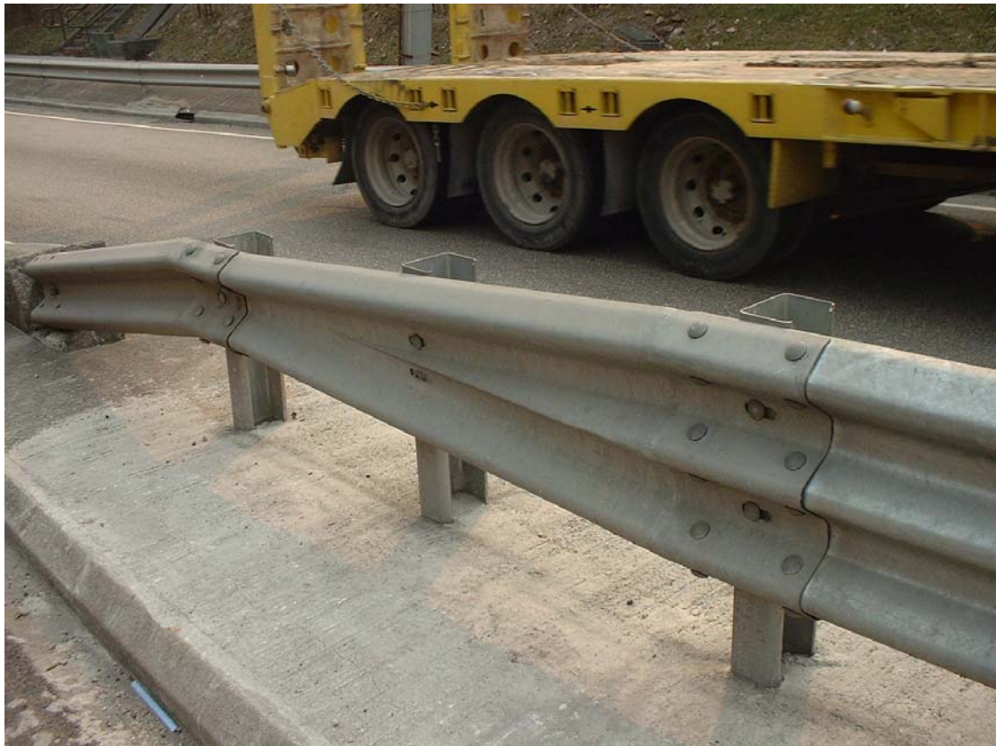
Photo 1: Existing Leading Terminal of Thrie-beam Barrier Fence at Roadside
