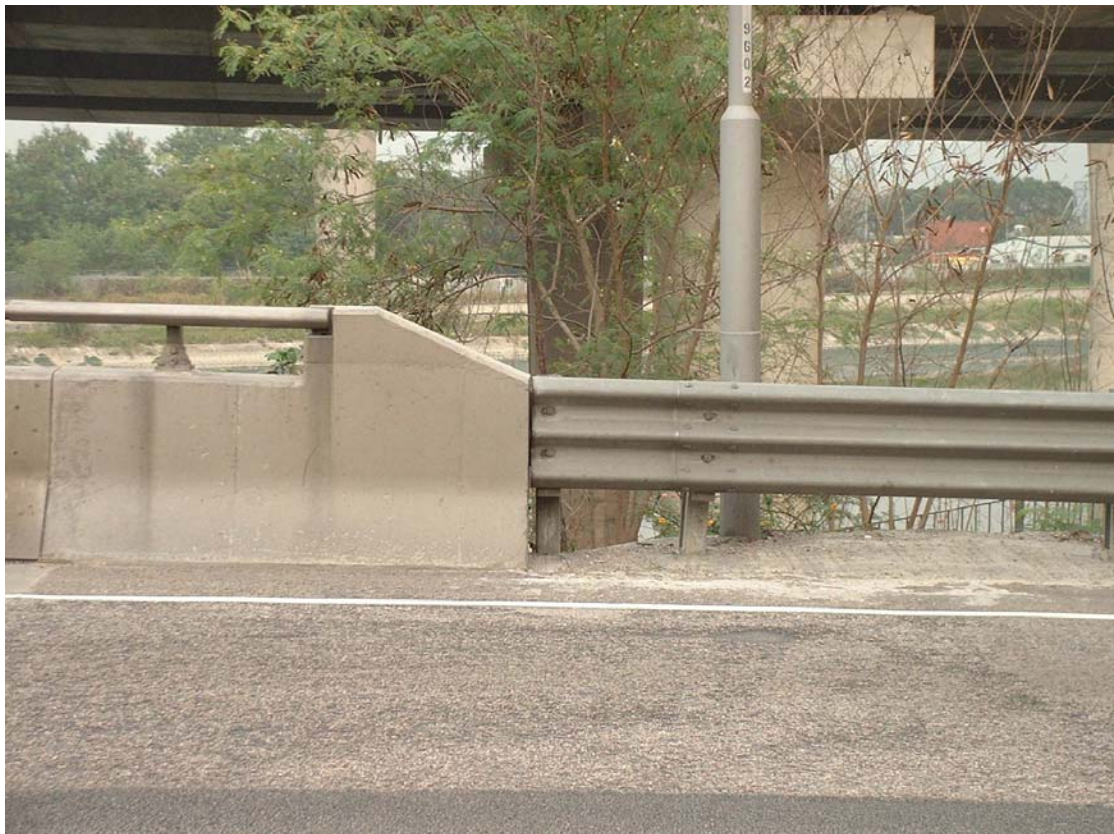
Photo 4: Existing connection of a Concrete Vehicle Parapet to Thrie-beam Barriers
