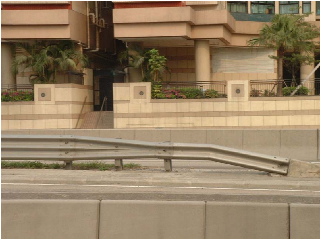
Photo 2: Existing Trailing Terminal of Thrie-beam Barrier Fence at Roadside.
