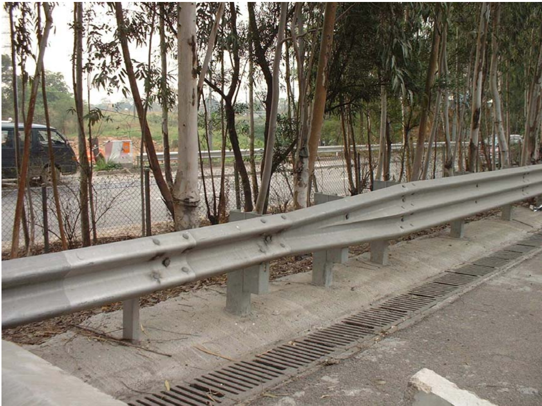
Photo 3: Existing Transition between Thrie-beam and W-beam
