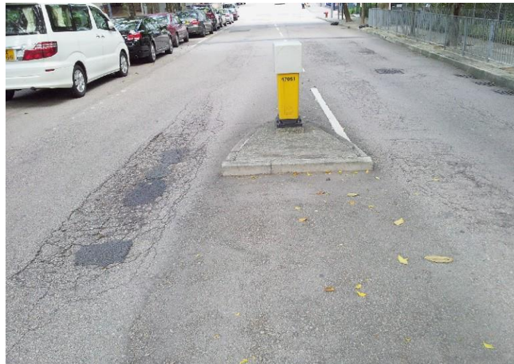
Photo 5 – severe surface distress requiring deep inlay
