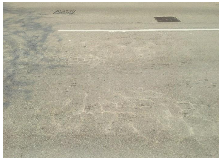
Photo 6 – sign of pumping from lean concrete base
