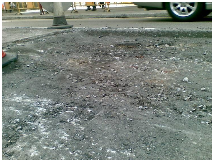
Photo 4 – Disintegrated base layer materials exposed after cold milling
