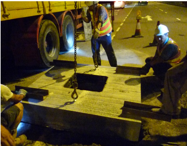
Two anchor bolts are used for lifting small panel
