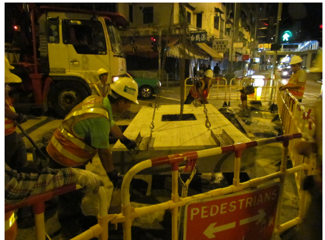
Four anchor bolts are used for lifting large panel
