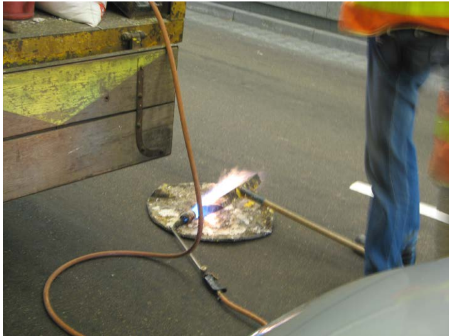
Plate No. 7 Heating up of Screed Box before Road Marking Application
