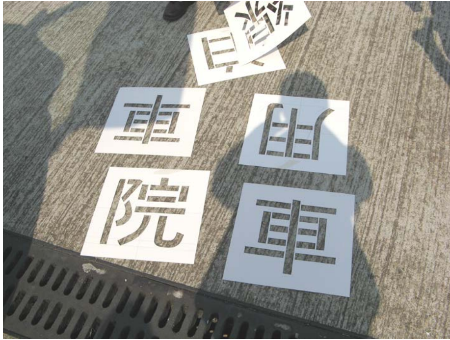
Plate No. 1 Use of Cardboard Molds for Marking of Symbols or Characters
