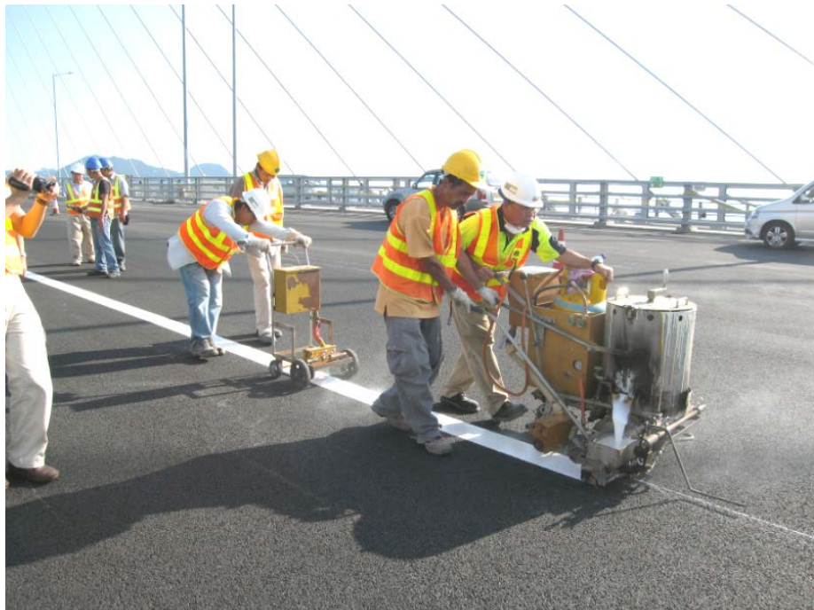
Plate No. 16 Combined Usage of Thermoplastic Screed Machine and Hand Push Trolley (Dispense of Glass Beads) in a Road Marking Operation
