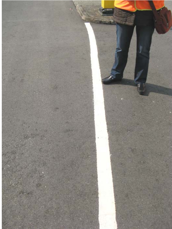
Plate No. 11 Improper Curved Lines Finished by Free Hand
