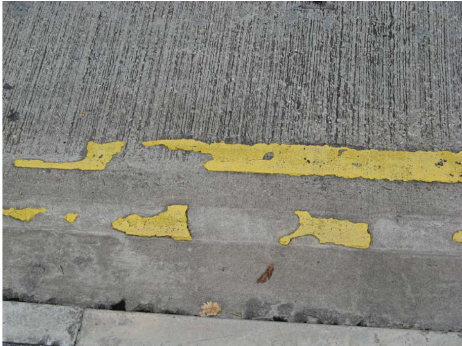
Plate No. 3 Flake off of Thermoplastic Material from Concrete Surface
