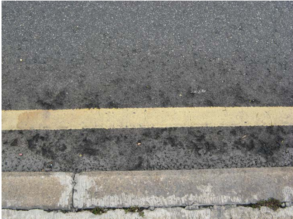
Plate No. 5 Discolouration of Yellow Road Marking
