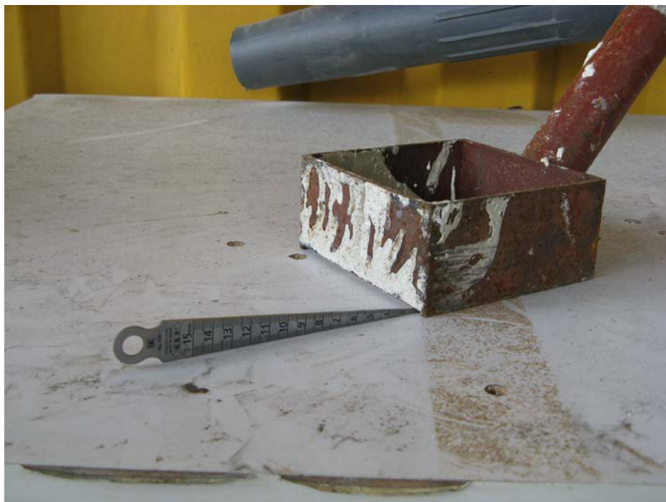
Plate No. 8 Height of Gap of the Screed Box Checked by Caplier
