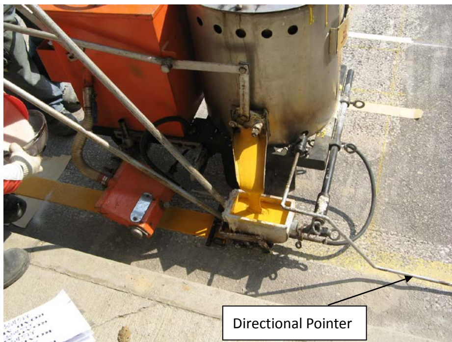
Plate No. 14 Close View of Directional Pointer of the Screed Machine
