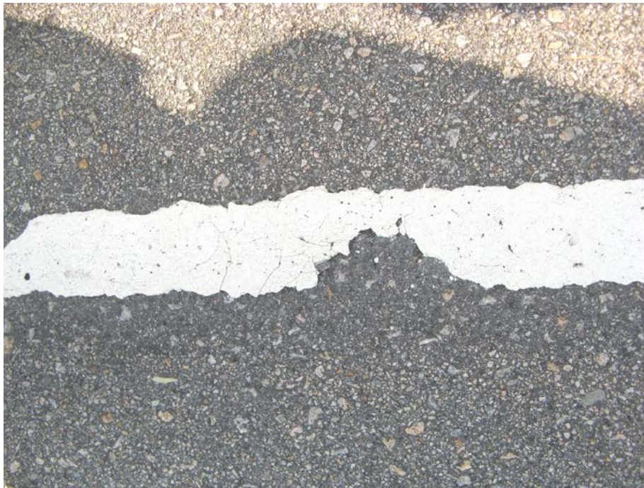
Plate No. 6 Early Detachment of Thermoplastic Material
