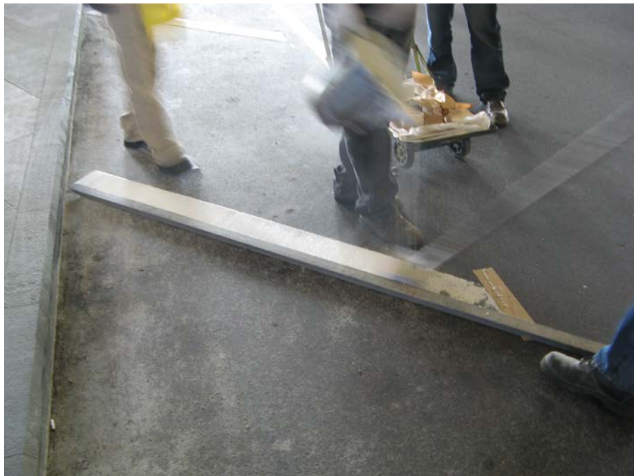
Plate No. 12 Use of Temporary Tapes at the End of Marking to Prevent Over-paint
