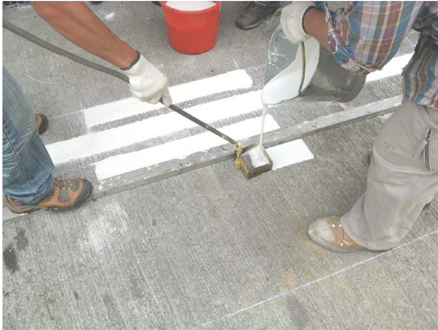
Plate No. 9 Use of Straight Edges for Line Marking
