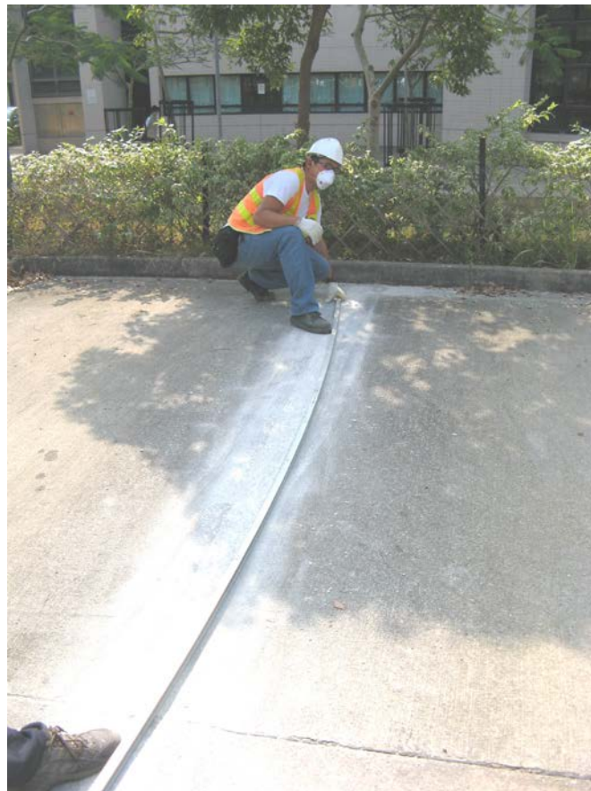
Plate No. 10 Use of Flexible Edge for Curved Lines
