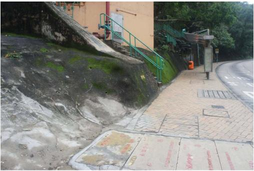
No interception channel at toe of the slope between the two natural streams
