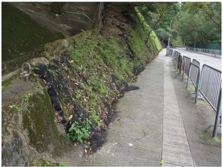
No interception channel along a short section of slope toe
