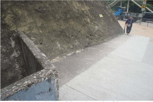
No interception channel along a short section of slope toe
