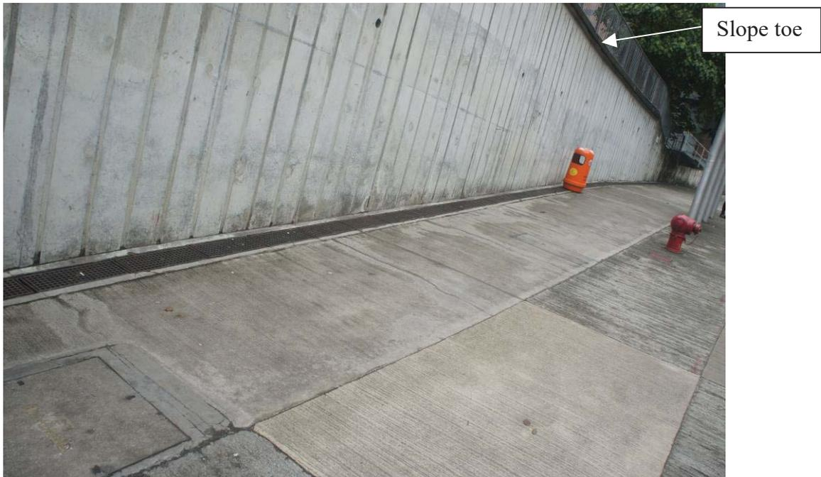
Retaining wall with interception channel at slope toe
