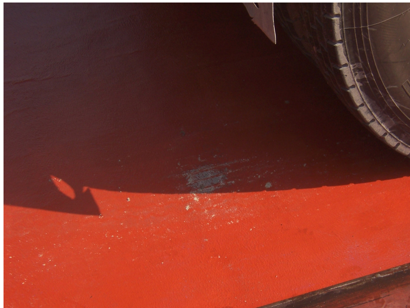
Photo 4 – Damage to the tack coat by the wheels of delivery trucks during laying mastic asphalt on a steel bridge deck of Shenzhen Western Corridor.
