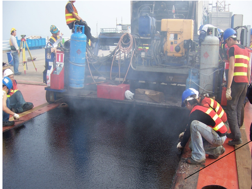
Photo 3 – Laying of mastic asphalt on top of polymer waterproofing membrane on a steel bridge deck of Shenzhen Western Corridor. To avoid damage to the tack coat and polymer waterproofing membrane, the paving machine rode on a protective layer laid on top of the tack coat.
