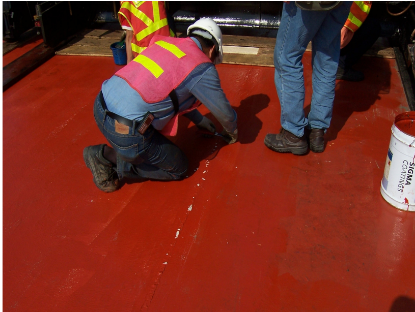
Photo 5 – The damage to the tack coat was made good by reapplying tack coat immediately.
