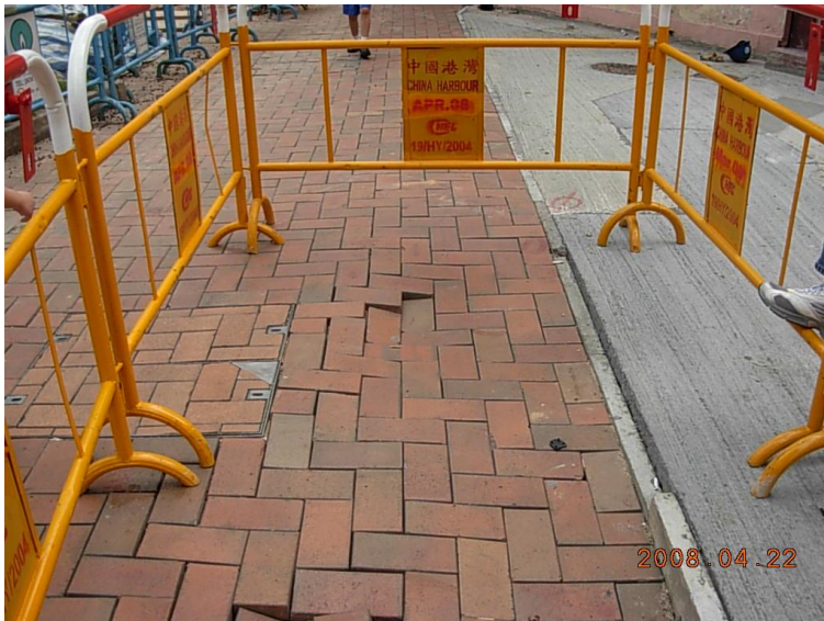
Plate 2: No proper boxing out of road slab was constructed around manhole covers (see Drg. H1111).
