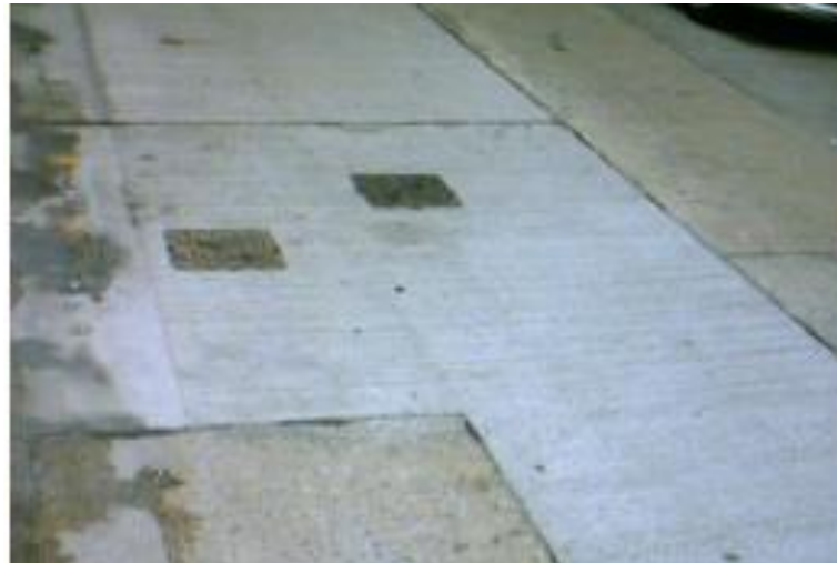
Plate 2: No proper boxing out of road slab was constructed around manhole covers (see Drg. H1111).
