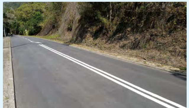
Rubberized bituminous pavement material laid at Bride's Pool Road
