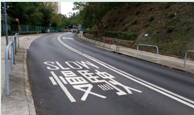
PMSMA6 laid at Tai Tam Road
