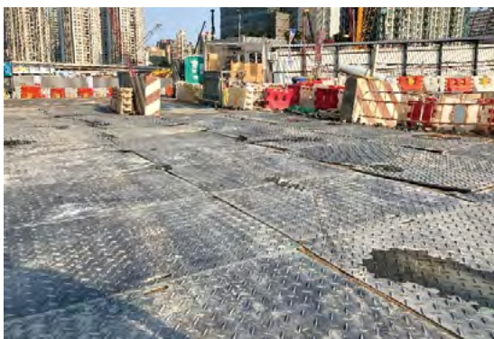
Use of recycled HDPE mats for site haul roads in Contract No. HY/2014/20
