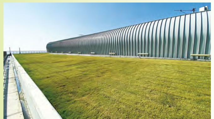
Rooftop greening at North Ventilation Building
