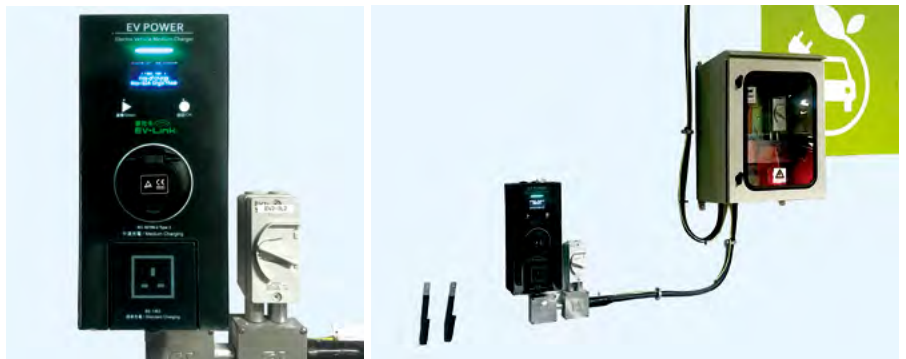
New 32A medium charger at Trade and Industry Tower
