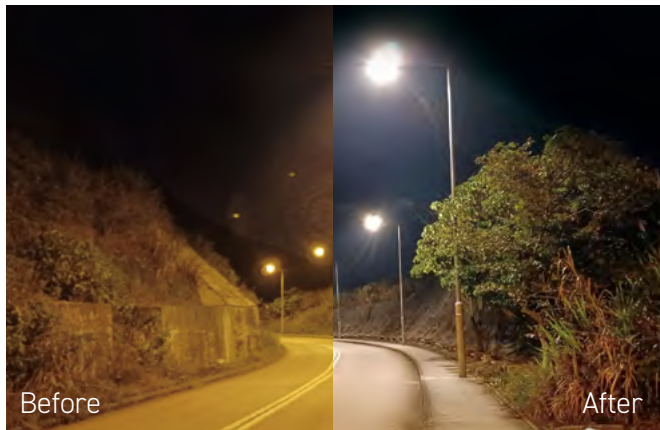
Conventional High Pressure Sodium lights at Tai Au Mun Road in Sai Kung
