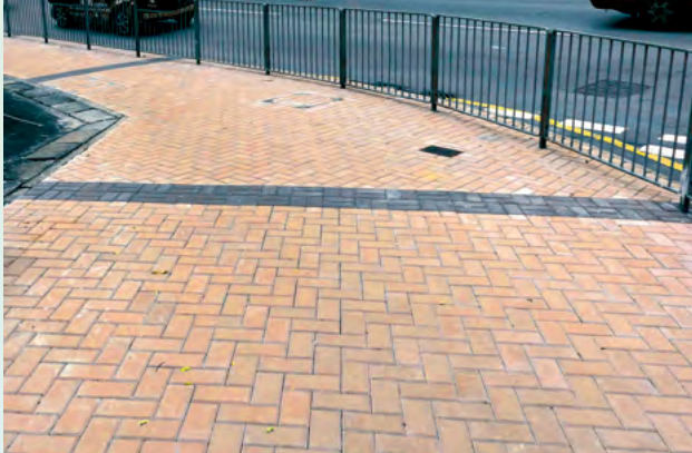
Site trial of eco-pavers at Tai Pak Tin Street, Kwai Chung
