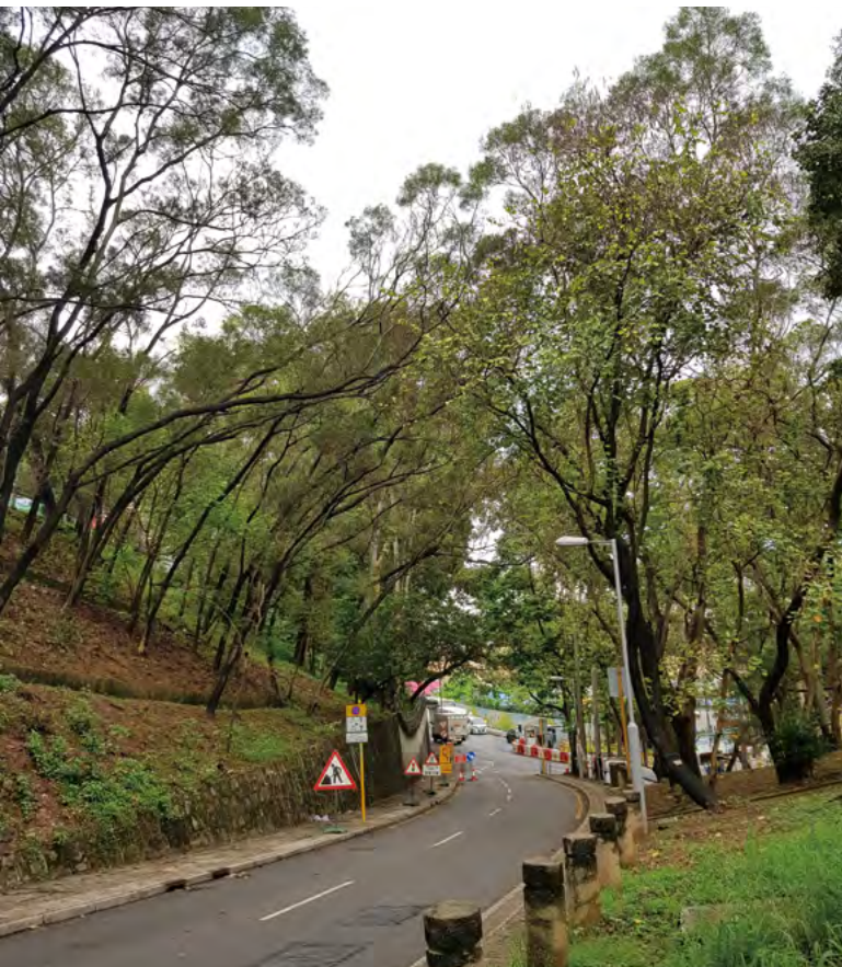
Trees on vegetated slope maintained by the Highways Department
