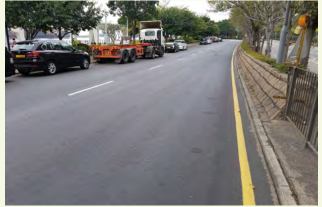
Rubberized bituminous pavement material laid at Hoi Fai Road
