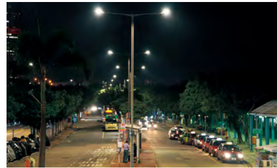
A public road with LED lights
