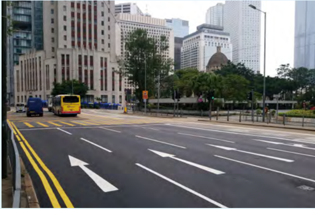
PMSMA6 laid at Queensway
