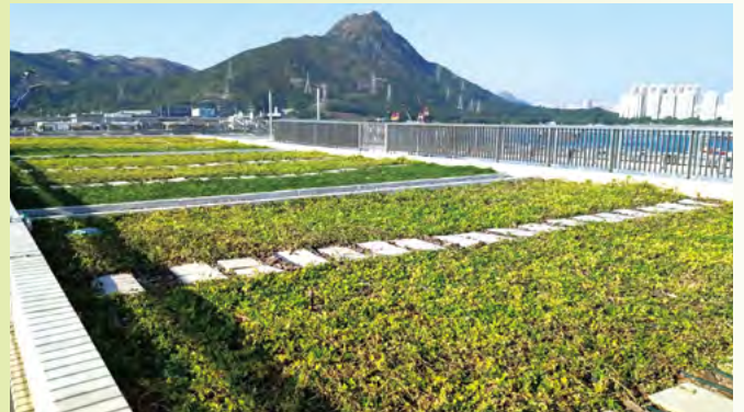
Rooftop greening at the Tuen Mun Customs Marine Base
