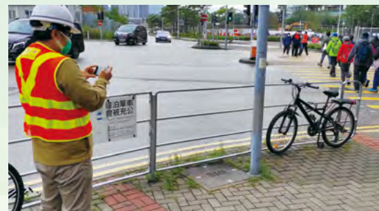
Engineer Inspection - unwanted vegetation
