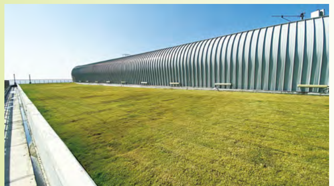
Rooftop greening at North Ventilation Building
