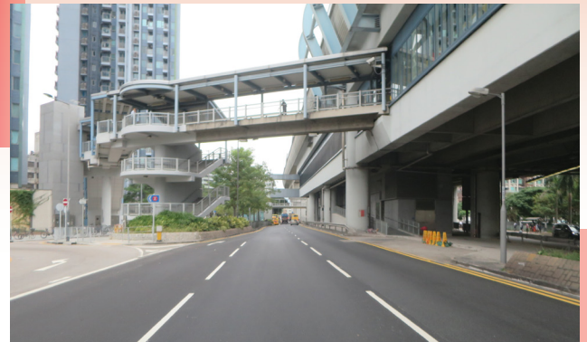
▲ PMSMA6 laid at Long Yip Road
