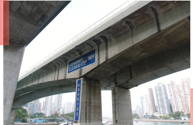
▲ Overview of Ap Lei Chau Bridge
