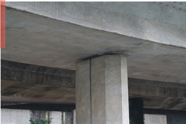
▲ Close-up view (column)
