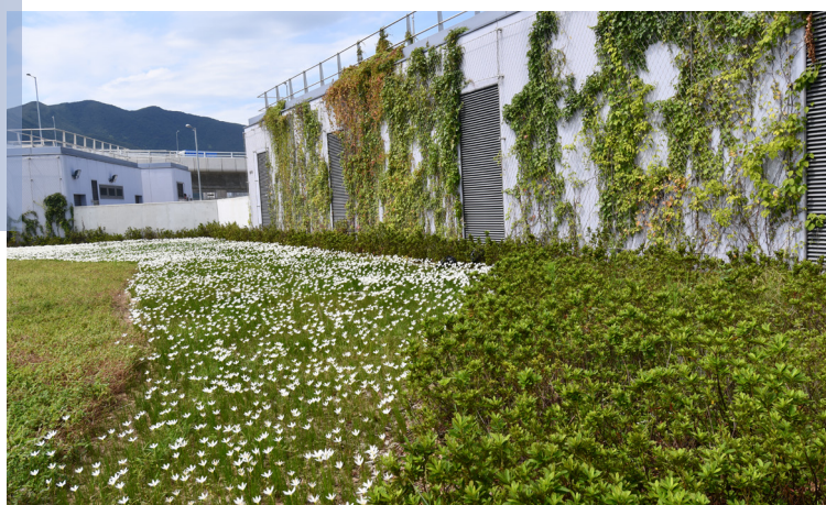
▲ Green roof and wall of the Fire Station cum Ambulance Depot
