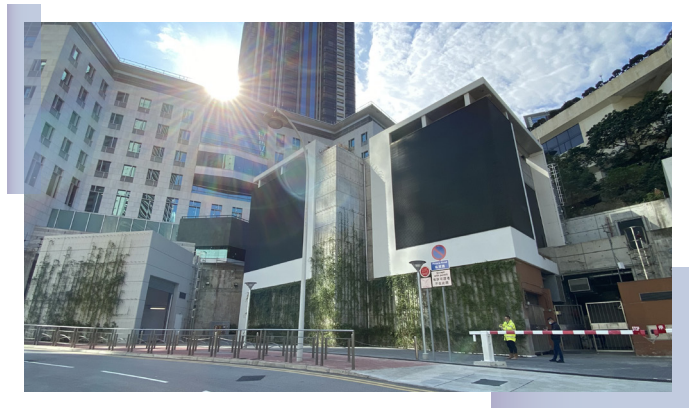
▲ Vertical greening at Hong Kong Park Ventilation Building
