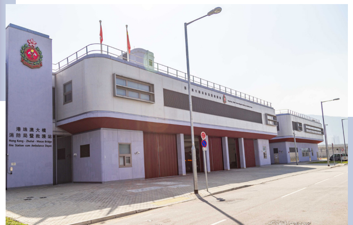
▶ The Fire Station cum Ambulance Depot
