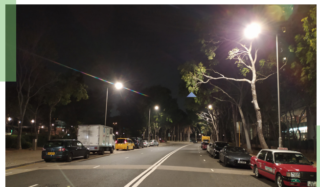
▲ Same location after replacement with LED lights
