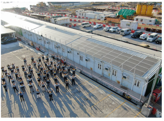
Solar panel on the roof of the site office of Contract No. HY/2014/07
