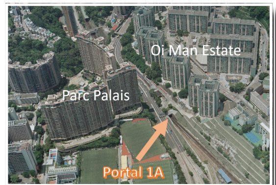
Location of tunnel portal 1A
