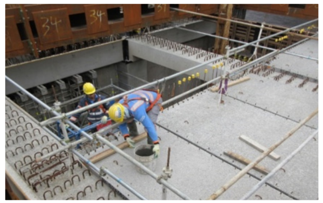
Installation of precast slabs
