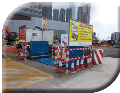
Provide wheel washing machine at site entrance
