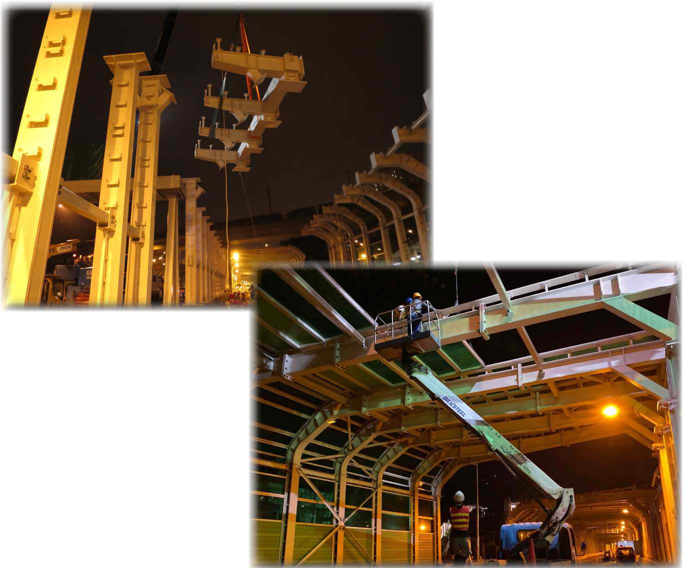
Erection of steelworks and installation of noise panels at night time
