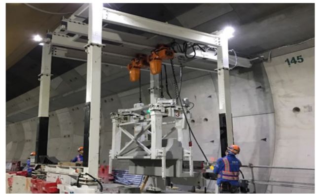
Installation of precast parapets
