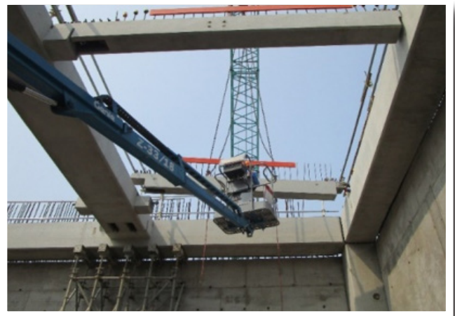
Installation of precast beams
