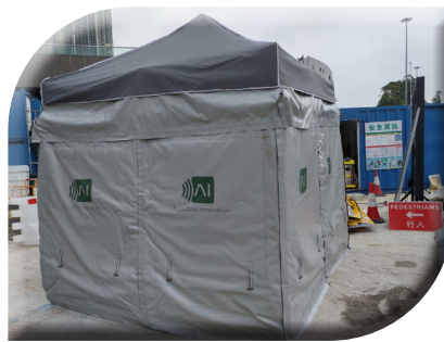
Cover plant with acoustic enclosure
