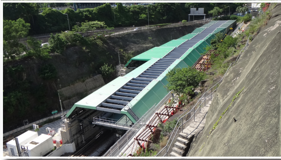
The completed noise enclosure at tunnel portal 1A near Oi Man Estate
