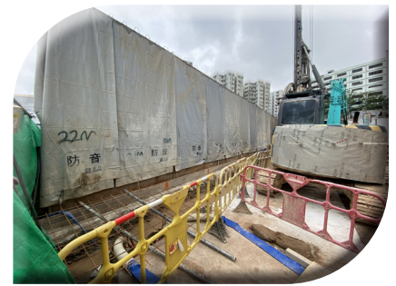
Erect acoustic fabric barriers
