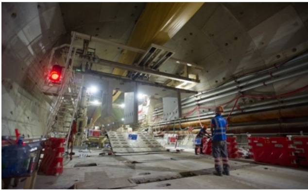
Installation of services galleries
