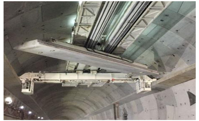
Installation of overhead ventilation duct slabs
