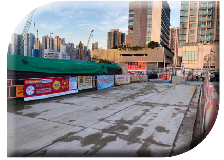
Use concrete plank as vehicle access for dust control
