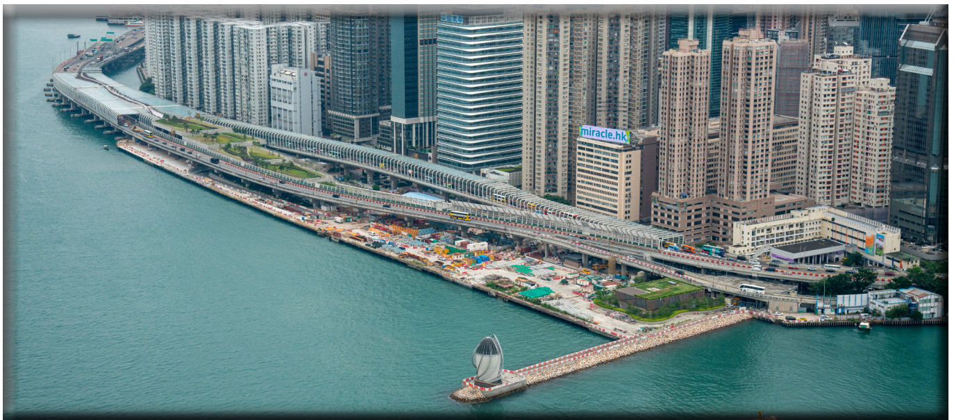
Noise enclosures and noise barriers on IECL
