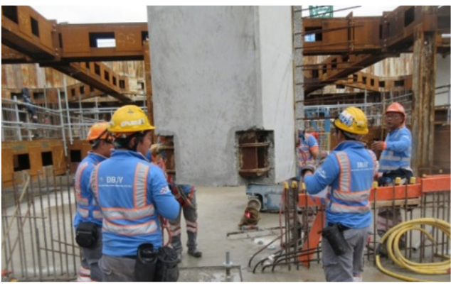
Installation of precast columns
