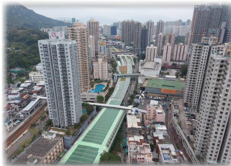
Noise barriers and enclosures on Tuen Mun Road (Town Centre Section)
