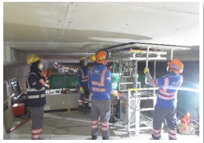
Installation of board-type thermal barrier
