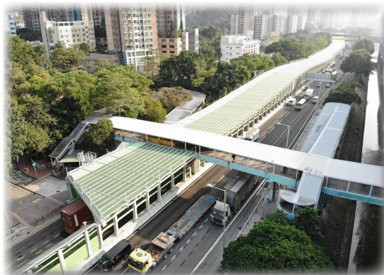
Noise barriers and enclosures on Tuen Mun Road (Fu Tei Section)
