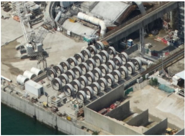
Precast jacking pipes for cross passages
