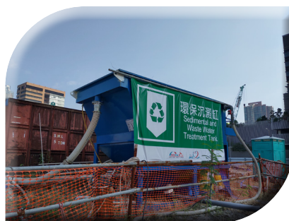
Use wastewater treatment facilities
