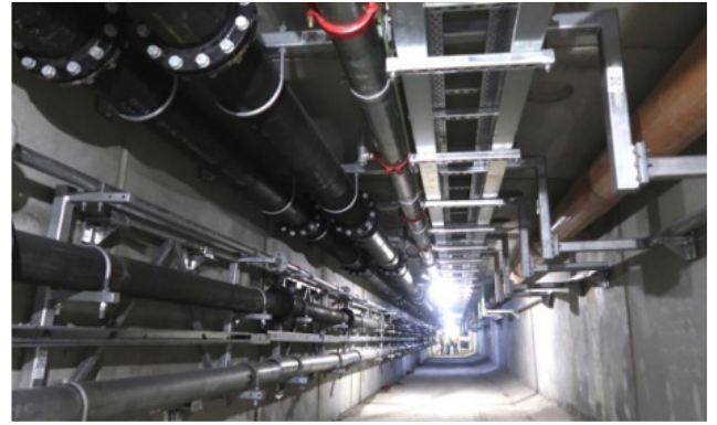
General view of completed services
