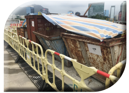
Collect scrap metal from piling works for recycling
