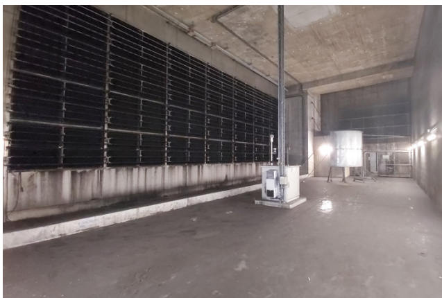
Electrostatic precipitators
