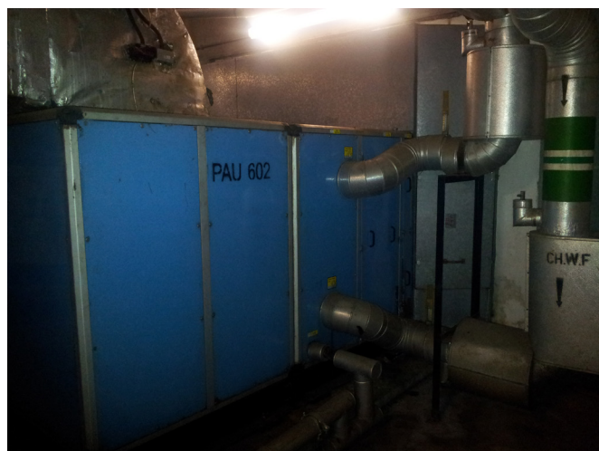
Replacement of the fresh air unit
