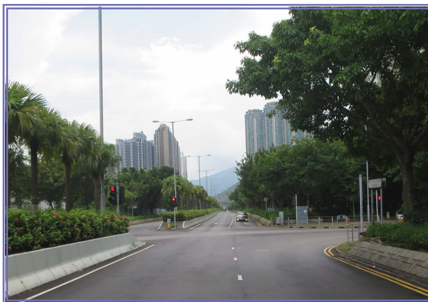
PMSMA6 laid at Tung Chung Waterfront Road
