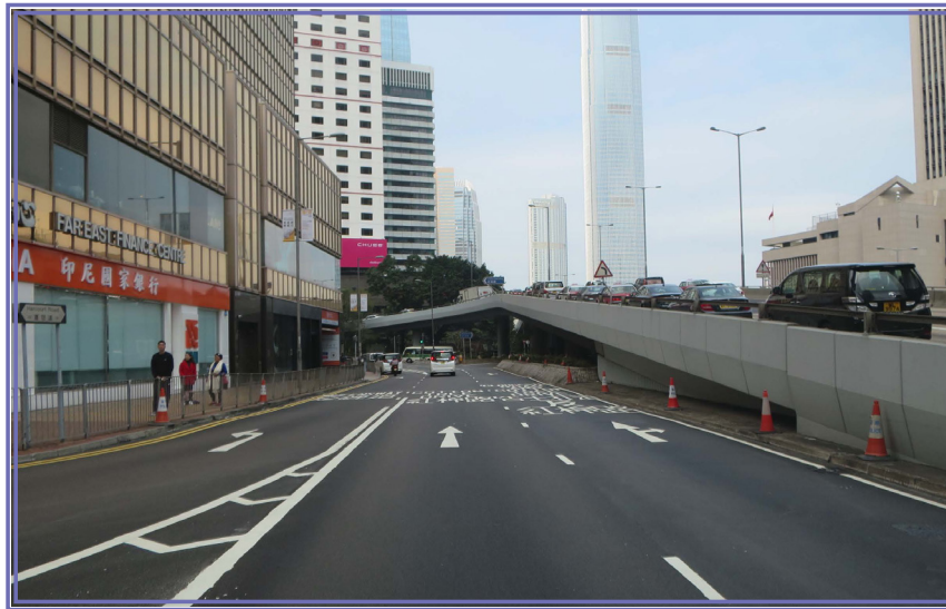
PMSMA6 laid at Harcourt Road
