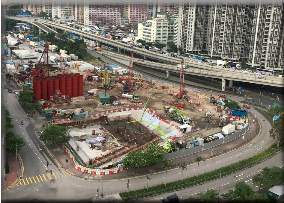
A construction site of the CKR
