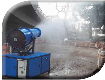
Suppress dust on haul road with water mist cannon
