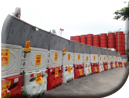
Erect acoustic fabric barriers along site boundary
