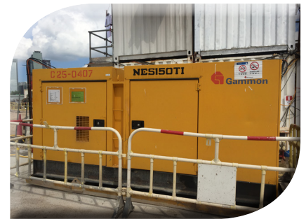
Use quality powered mechanical equipment to reduce noise impact
