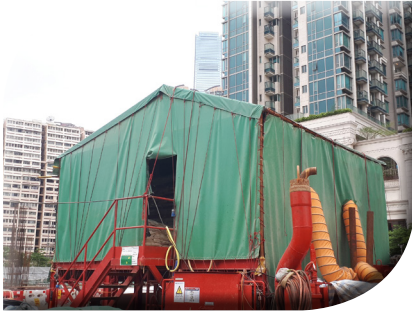
Set up full enclosure for controlling dusty activities
