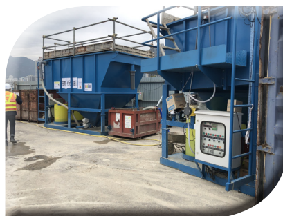
Use wastewater treatment facilities
