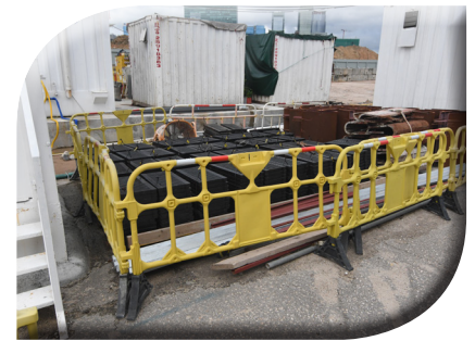
Implement good housekeeping on site
