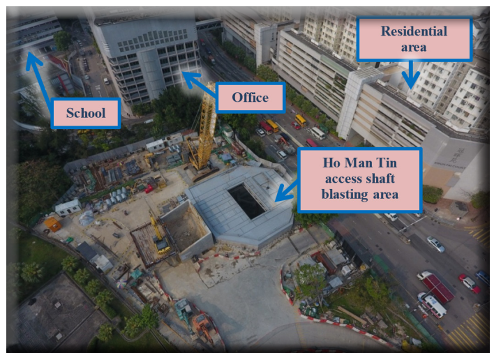
Noise enclosure at Ho Man Tin construction site
