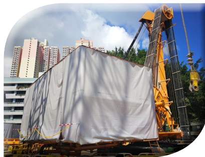
Cover plant with acoustic fabric for noise mitigation
