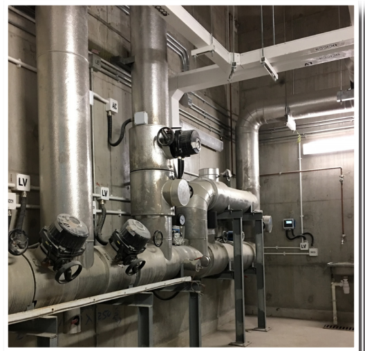
DCS substation in Kai Tak Station
