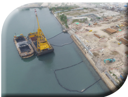
Deploy silt curtains during marine works
