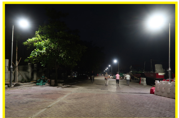
Peng Chau - After replacement by LED lights
