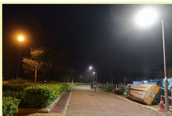
Peng Chau - Conventional High Pressure Sodium lights
