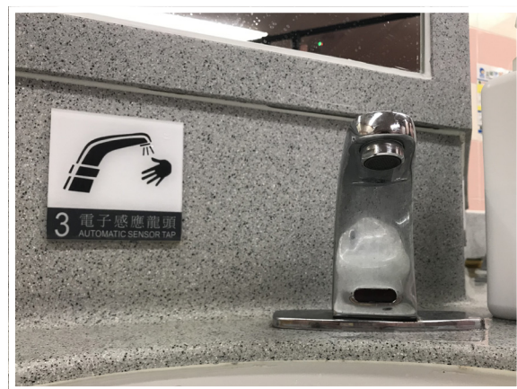
Installation of flow regulators for water saving
