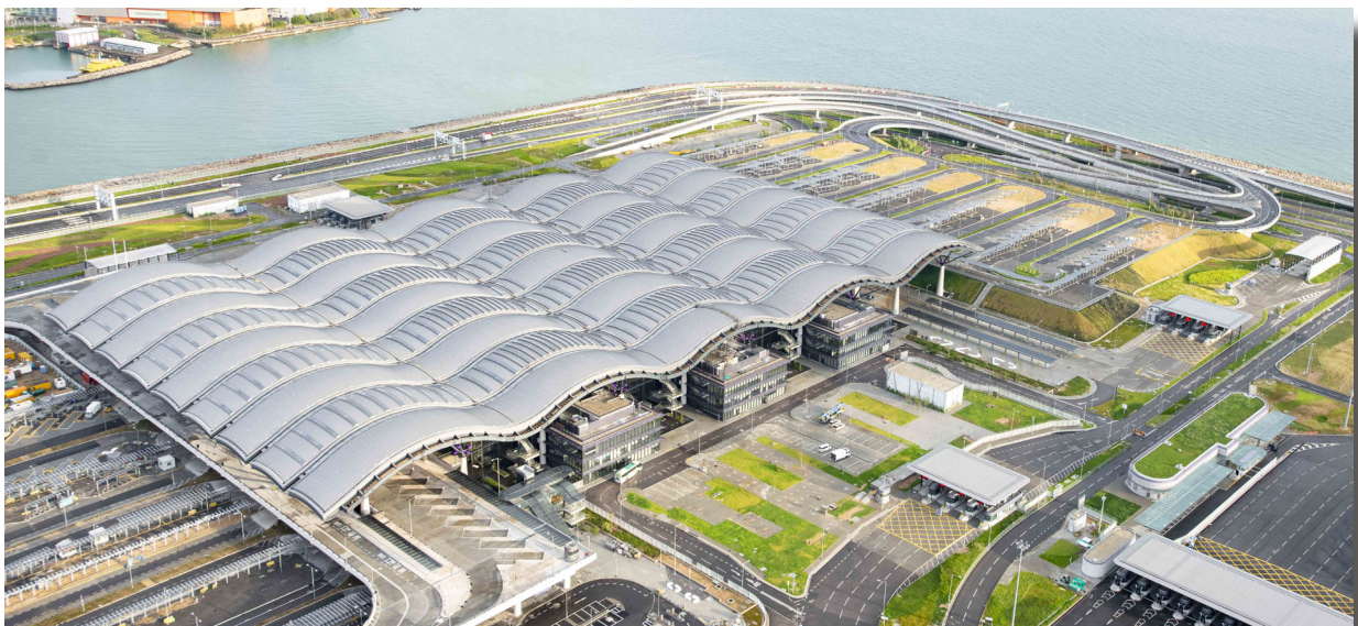
Roof of Passenger Clearance Building
