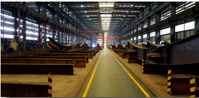
Fabrication yard for roof modules in Shaoxing
