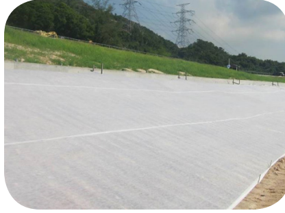
Carry out hydroseeding to exposed slope to suppress dust
