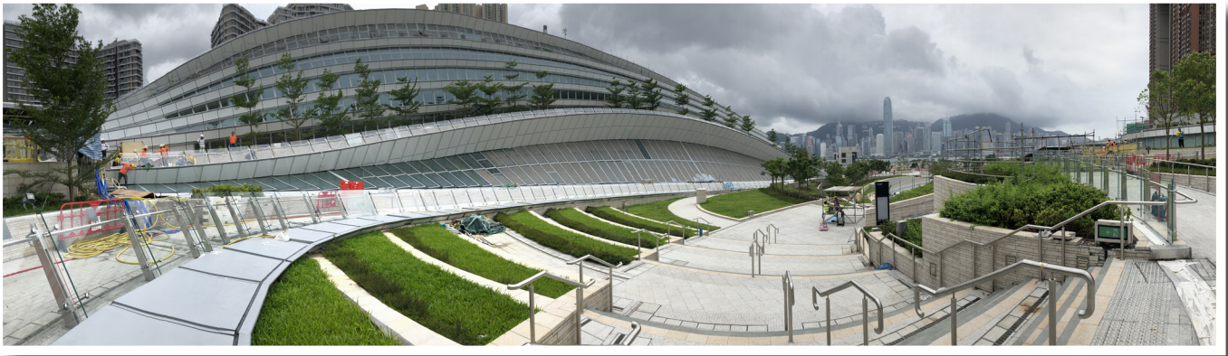
West Kowloon Station
