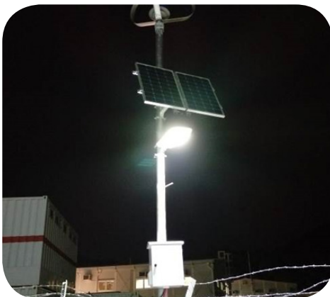
Install LED lighting with solar and wind energies for energy saving
