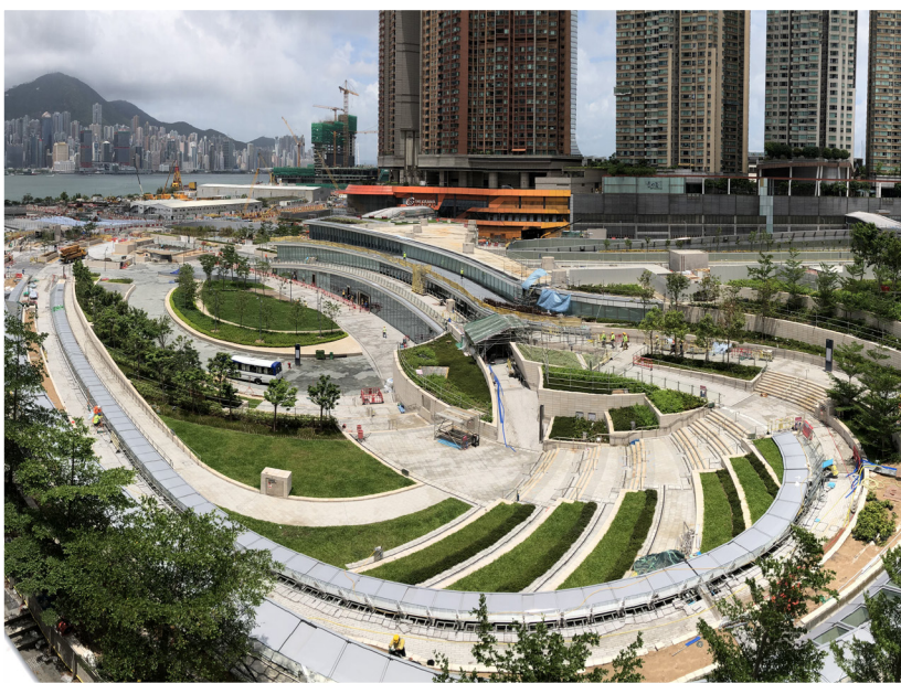
General view of West Kowloon Station
