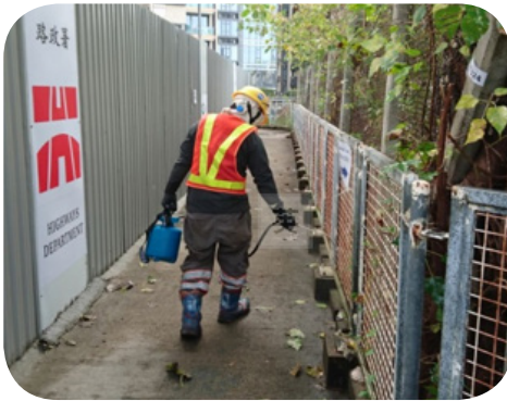
Prevent mosquito breeding near site
