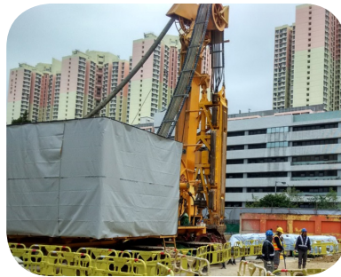
Cover plant with tarpaulin for noise mitigation control
