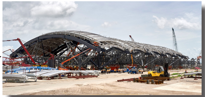
Assembly of roof modules in Zhongshan
