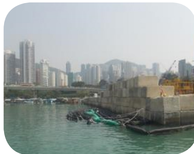
Deploy silt curtains during marine works
