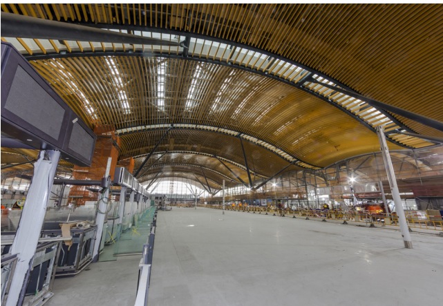
Skylights at roof (internal view)
