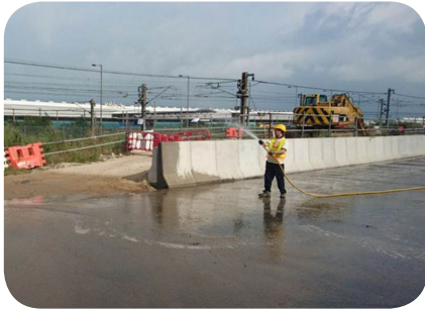
Spray water regularly on haul road to suppress dust
