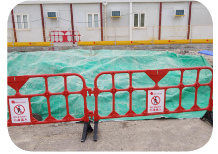
Cover exposed surface to control dust
