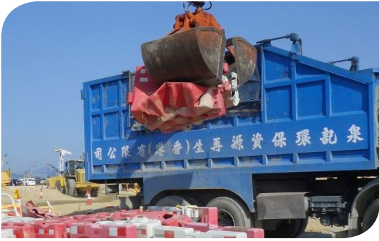
Recycle damaged water-filled barriers
