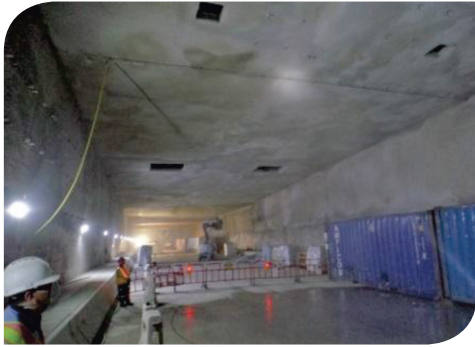
Water curtain system to prevent dust leaving the tunnel during spraying thermal barrier
