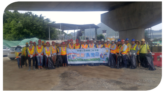
Organize regular site cleaning activity to promote good housekeeping on site
