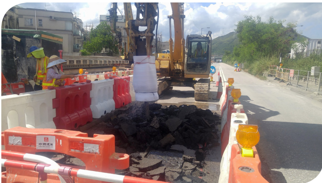
Wrap the breaker with sound absorption material
