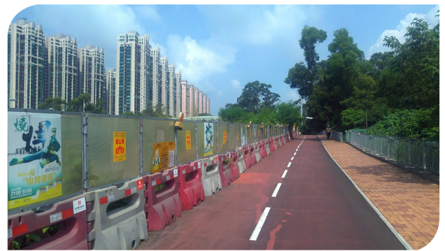
Erect plastic screen
