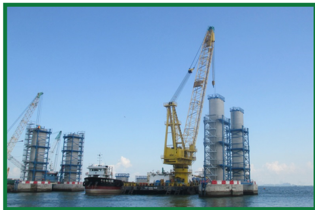
Construction of bridge piers at Western Waters of Hong Kong
