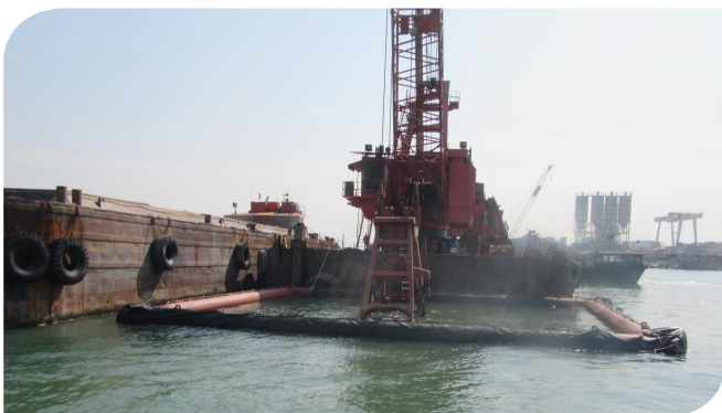
Use cage type silt curtain to mitigate impacts on water quality
