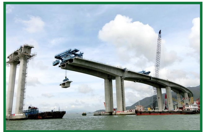
Installation of precast bridge deck segments at Western Waters of Hong Kong
