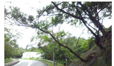
Acacia exhibits deteriorating health and declined structural conditions
