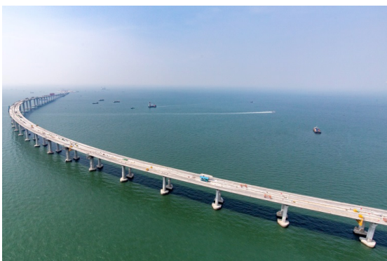
Aerial view of Marine Viaduct at Western Waters of Hong Kong
