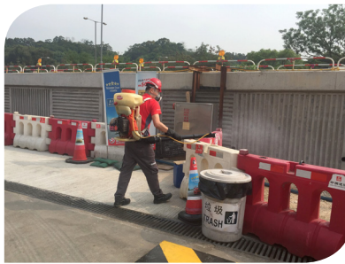
Pest control on site
