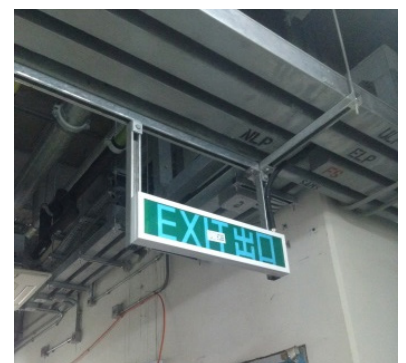
LED exit sign in Hin Keng Station
