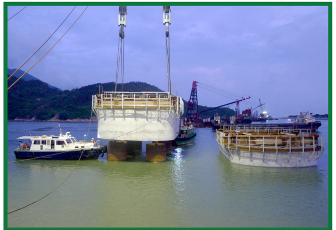
Installation of pile cap shell at Airport Channel
