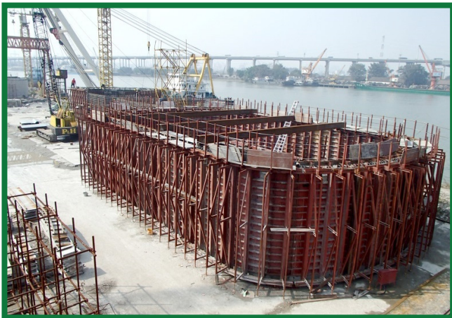
Casting of pile cap shells at Panyu, Guangzhou
