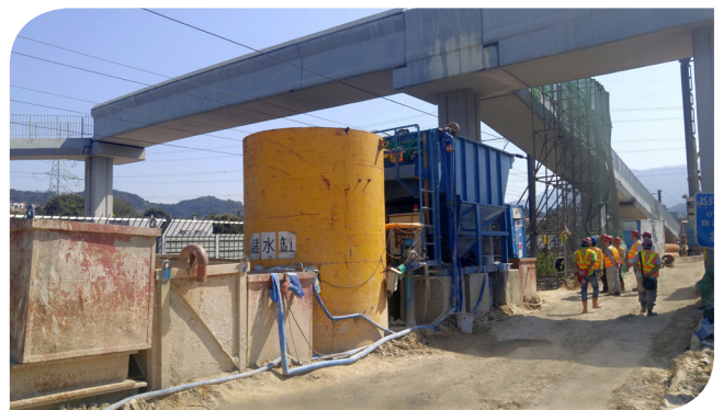
Wastewater treatment on site before discharge
