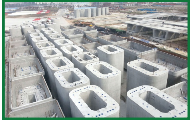
Bridge pier segments casting yard at Zhongshan
