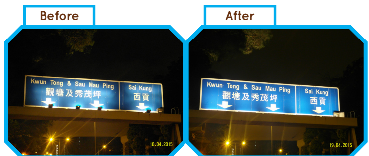
Gantry signs before and after the use of LED linear washer lights
