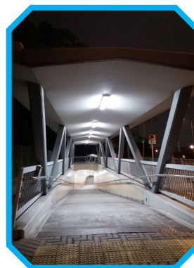
LED lights to replace T8 fluorescent tubes at subways
