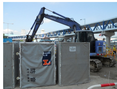
Movable noise barriers shielding construction noise
