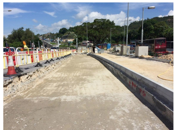
The surface condition of recycled aggregates after compaction
