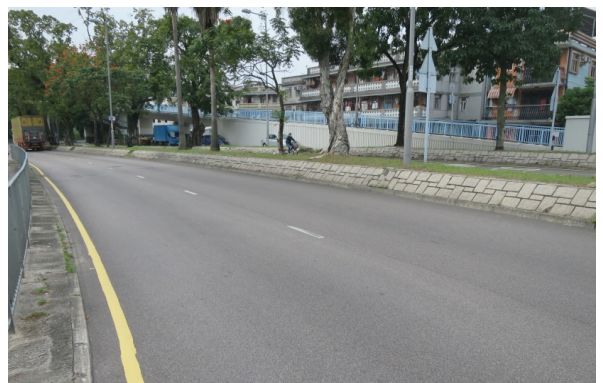
“Thin surfacing” at San Wan Road
