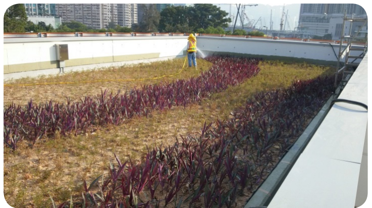
Green roof on ventilation building
