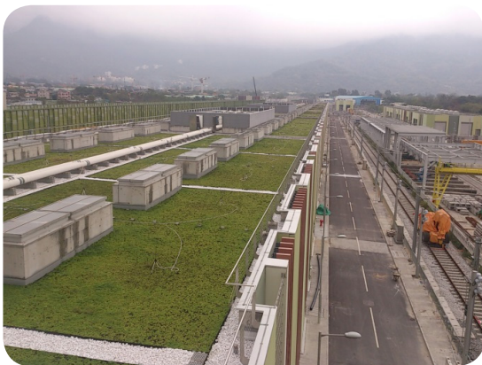
Green roof on maintenance shed in Shek Kong
