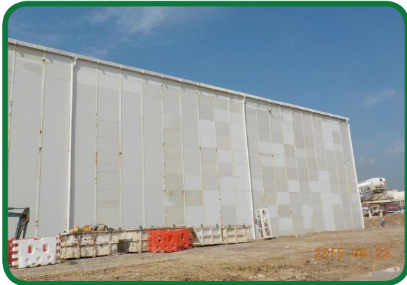
Noise Pollution Abatement – Noise enclosure at Slurry Treatment Plant
