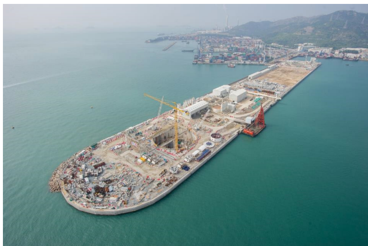
Aerial view of Northern Landfall
