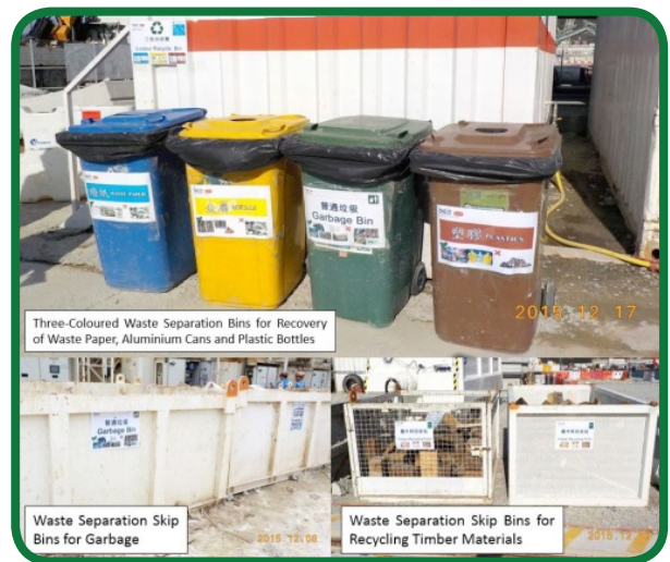
Waste Management – Segregation of different types of waste for recycling
