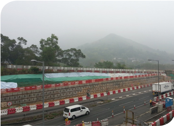
Cover the bare slope to prevent dust
