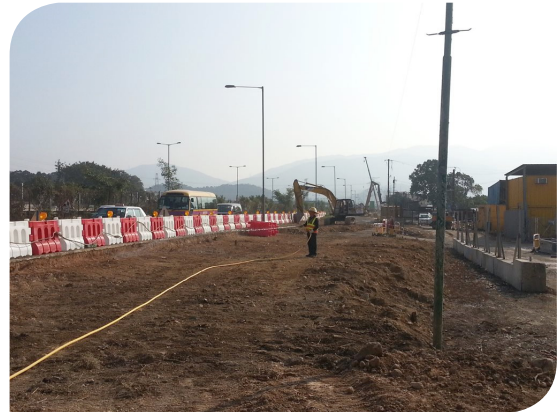
Spray water on exposed surface to prevent dust
