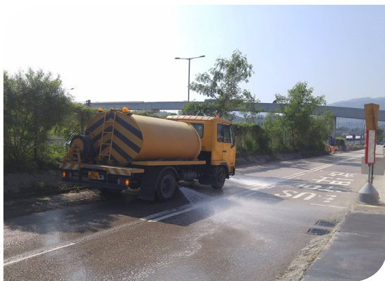
Wash the public road adjacent to the Site frequently
