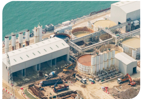
Recycle/reuse TBM spoil material
