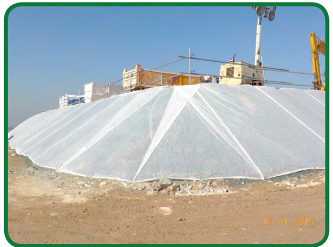
Air Pollution Abatement – Hydroseeding for surcharge slope to prevent dust dispersal
