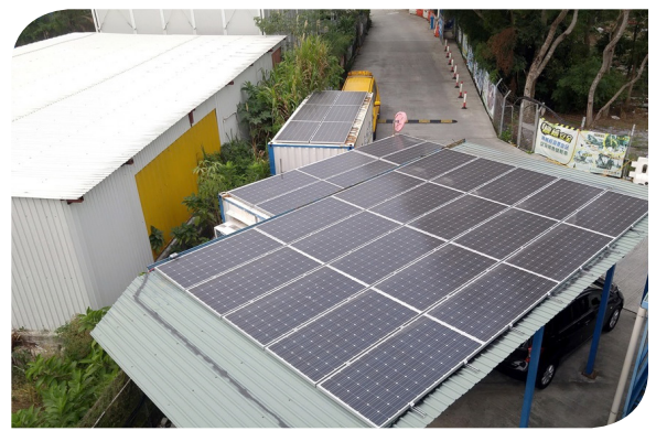
Install solar panel at site office compounds
