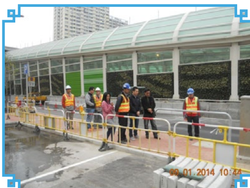
Site Visit with DC Member for the Reinstatement Works near Tsing Wu Square
