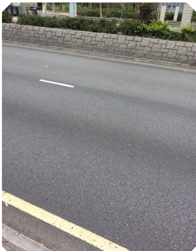
PMSMA Surfacing at Sha Tau Kok Road
