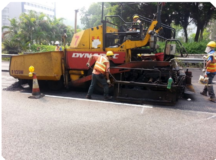
Resurfacing Works at Yu Tung Road, Tung Chung
