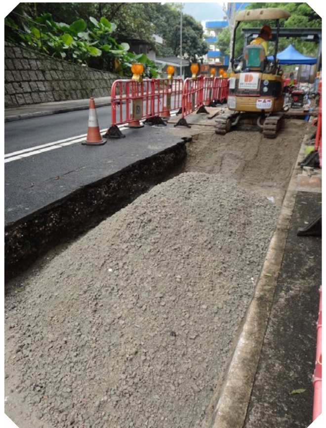
Laying Recycled Aggregates as Sub-base in Trial Site
