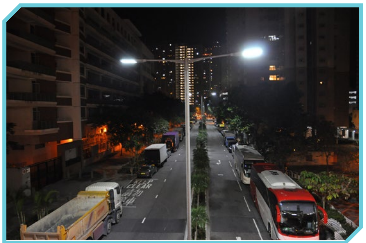
LED Road Lights
