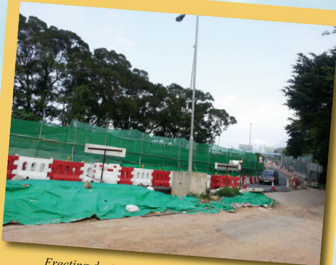
Erecting dust screen alongside works area
