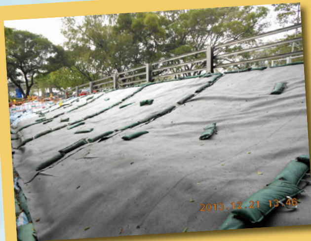
Covering the dusty materials with tarpaulin sheet
